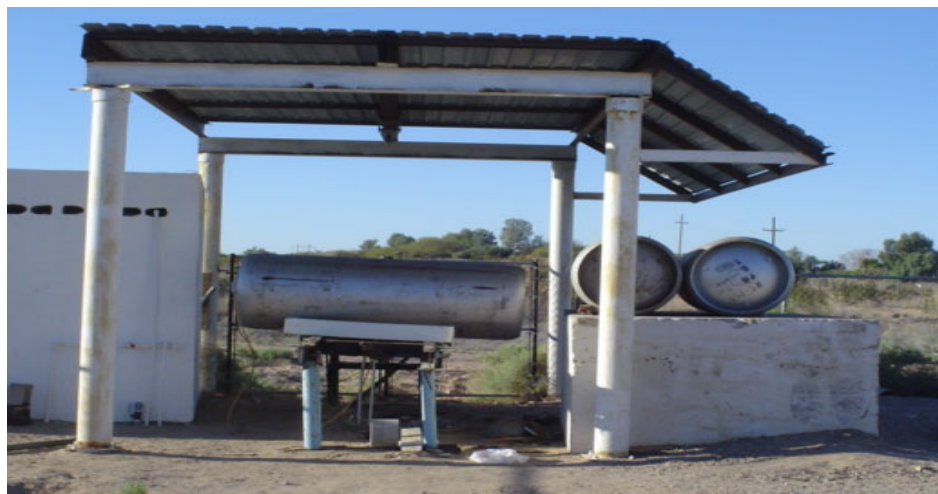
Notice the containers and see that these are not secured from rolling.
