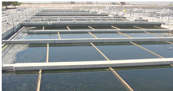
Rectangular Secondary Clarifier
