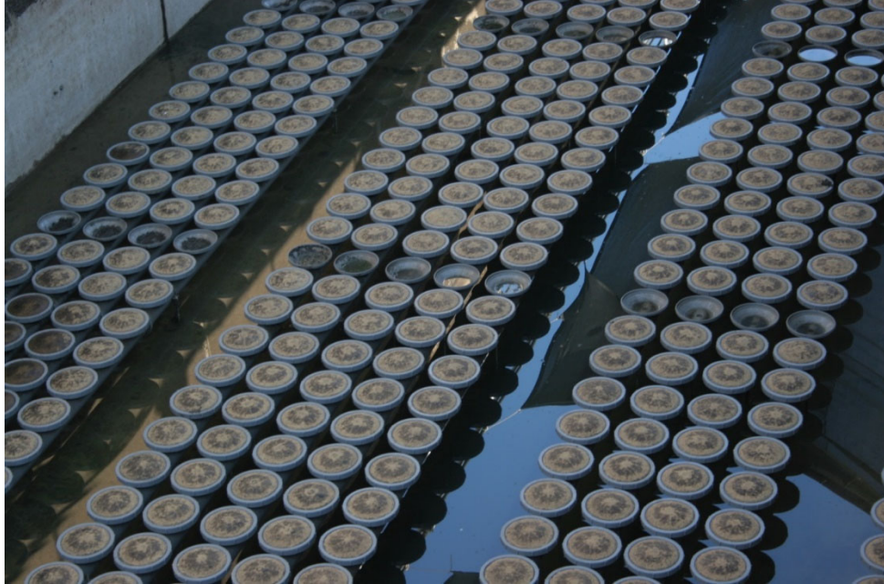
A up-close view of non-porous diffuser heads . Notice that some of the heads that are missing in the bottom photograph.
