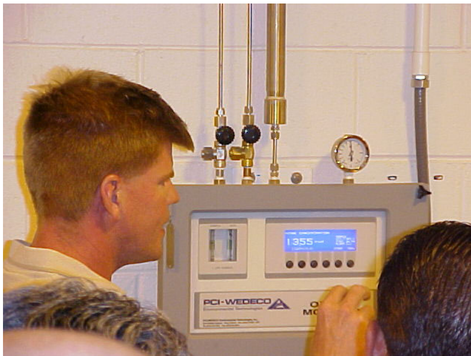
Ozone generator and control panel.
