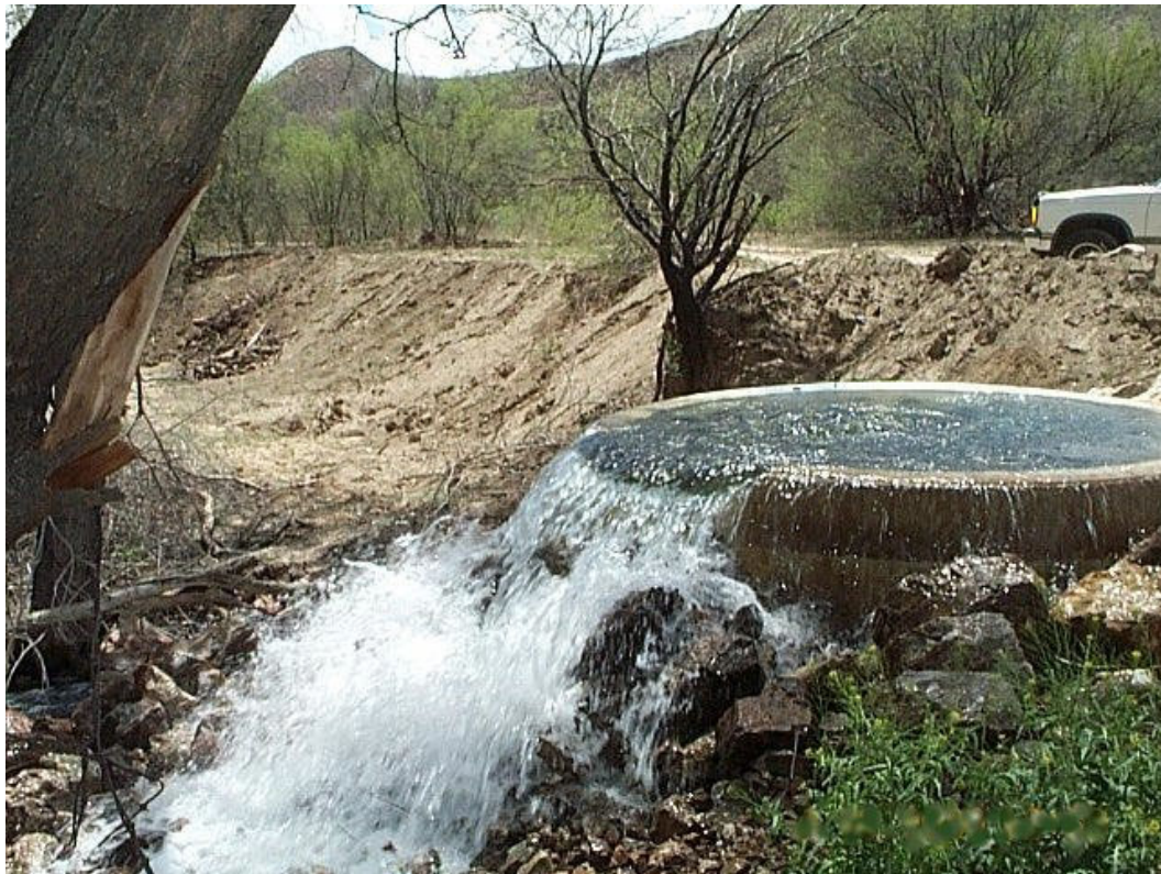
Treated wastewater outfall.
