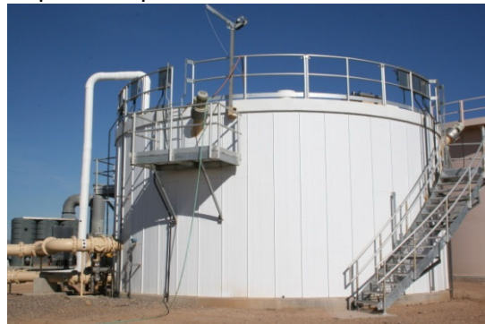
Anaerobic Digester
