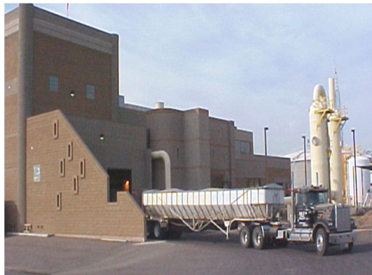
Large solids handling facility
