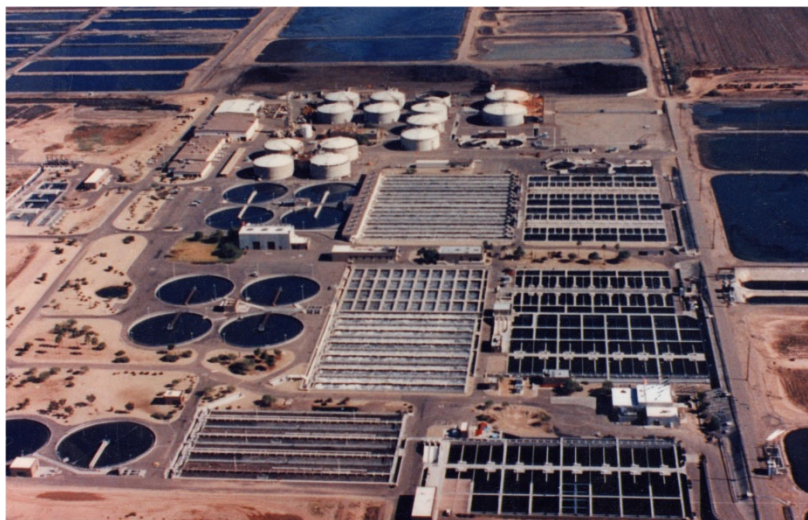
Modern wastewater treatment plant
