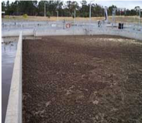
Figure 3. Dry Microthrix parvicella foam trapped in an anoxic zone of a BNR plant aeration basin.
