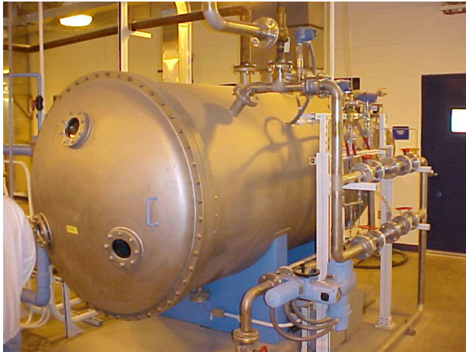
Ozone generator and control panel.
