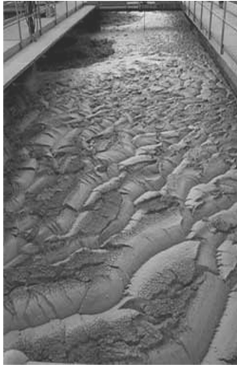
Figure 6. A heavy build-up of trapped Microthrix parvicella foam during winter.
