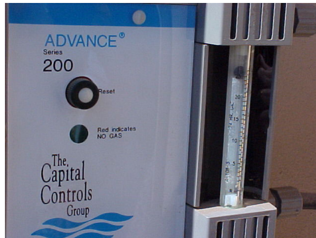
Chlorine measurement devices or Rotometers.
