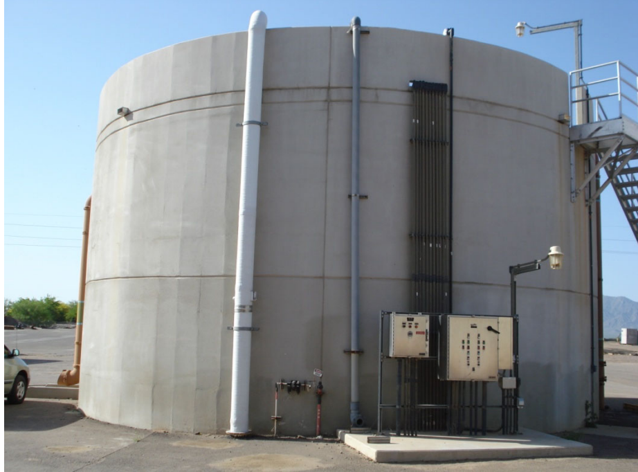
This clarifier is used to thicken sludge prior to the digester. This is not a digester but looks like one: Notice the light on the top for Operators to look inside.
