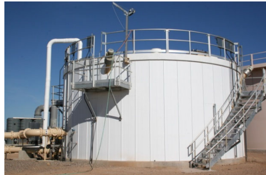
Anaerobic Digester
