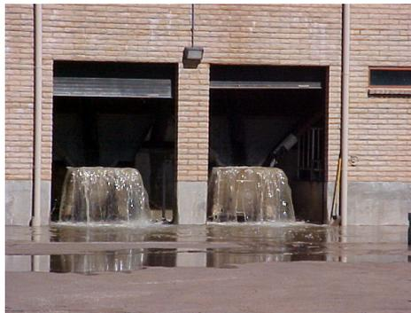
Domestic waste overflow at a WWTP headworks. Sometimes headworks do overflow, usually due to rags, grease and debris, or operator error. We do not like to see this happening!
