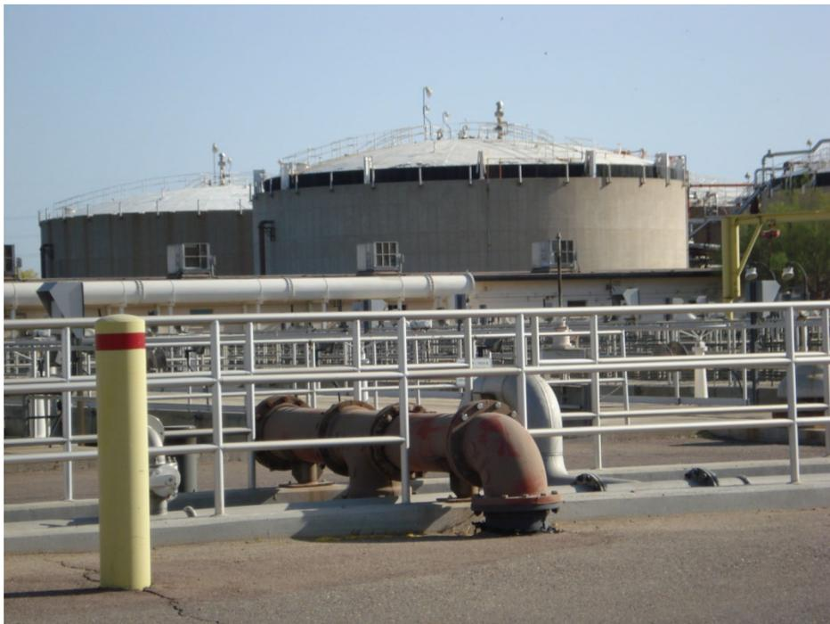
These two above ground circular tanks are massive anaerobic digesters.
