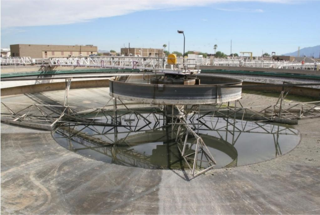
Top photograph, a clarifier's raking mechanism.
