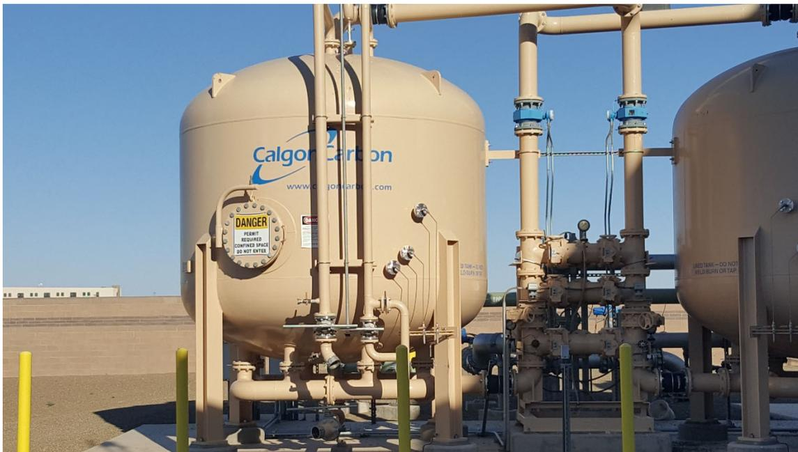
Granular Activated Carbon (GAC) vessel
