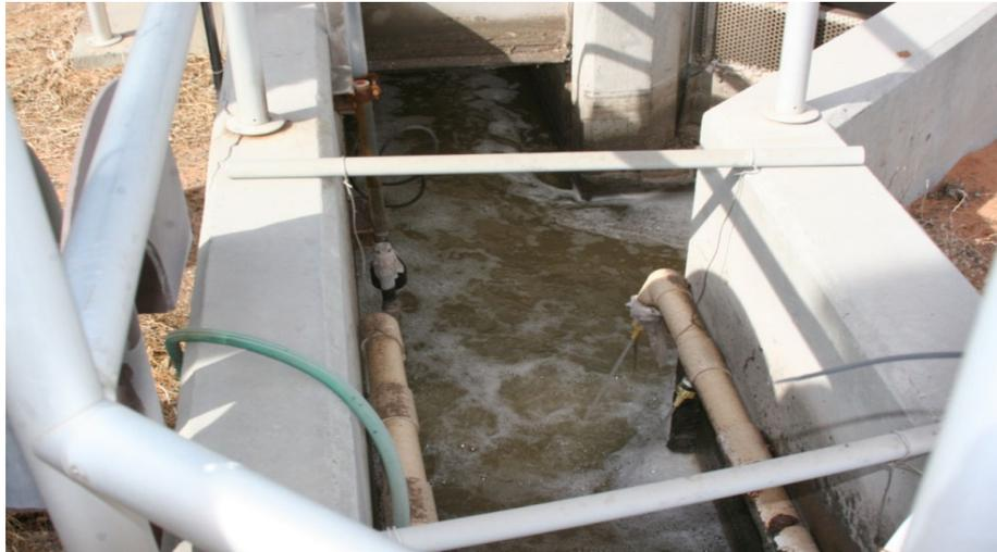
Aeration is often used to oxygenate the wastewater flow at the influent channel.
