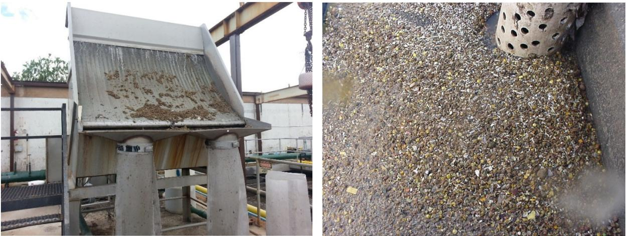
Left, Strainer Screen, Right, Floating debris in an influent wetwell
