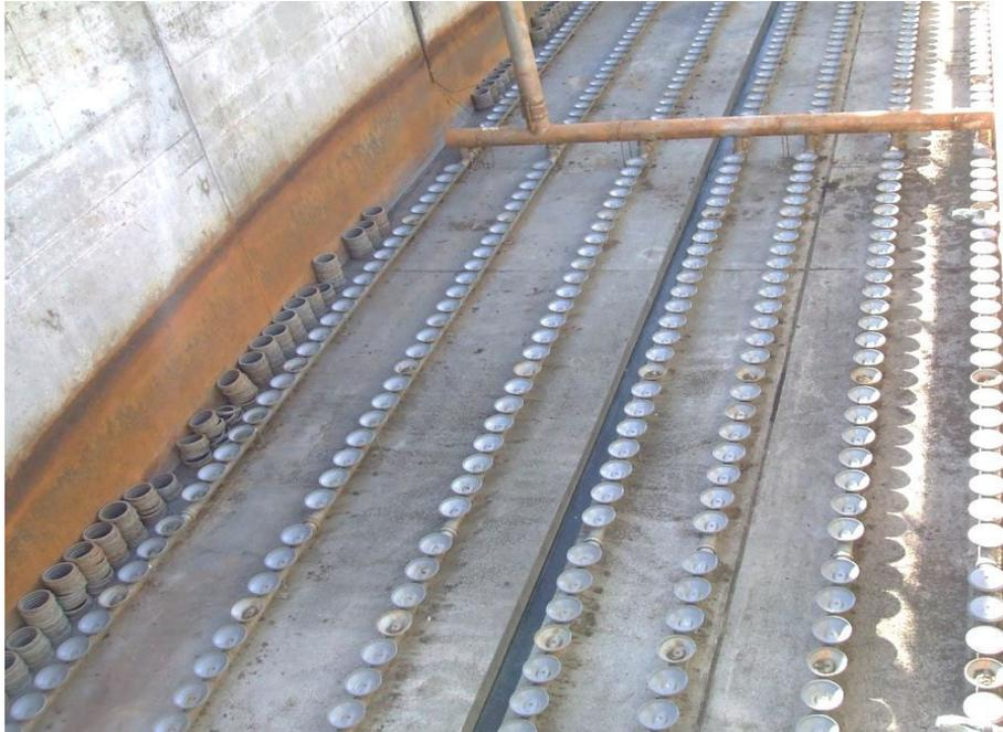
Porous air diffusers in an aeration tank.
