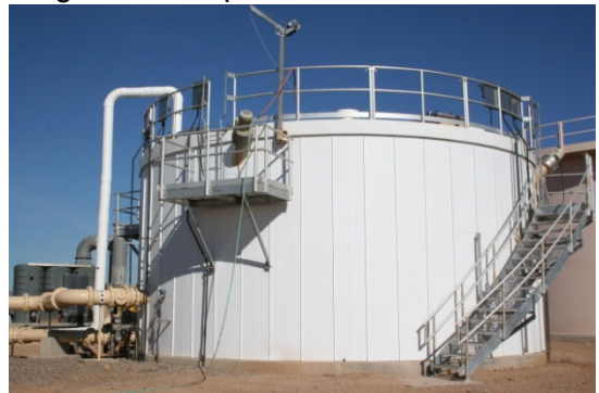
Anaerobic Digester
