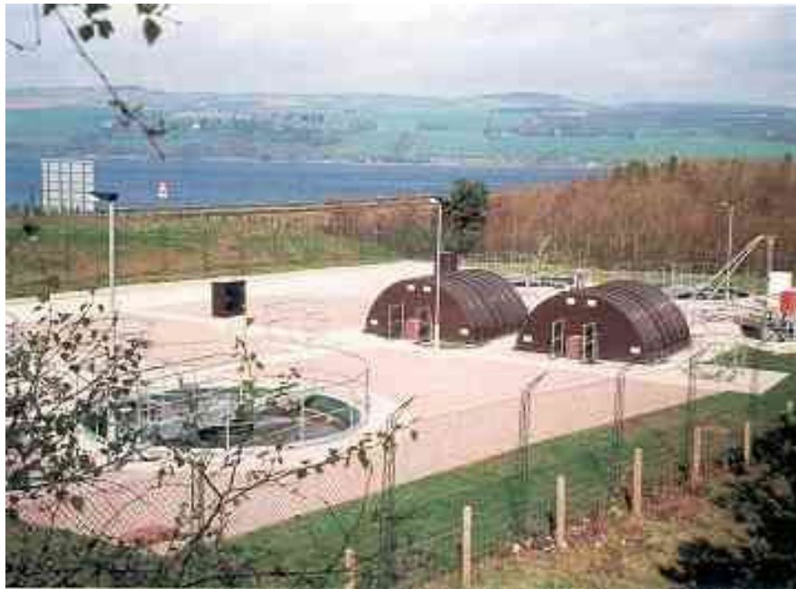
RBCs at Culbokie, Scotland Water.
