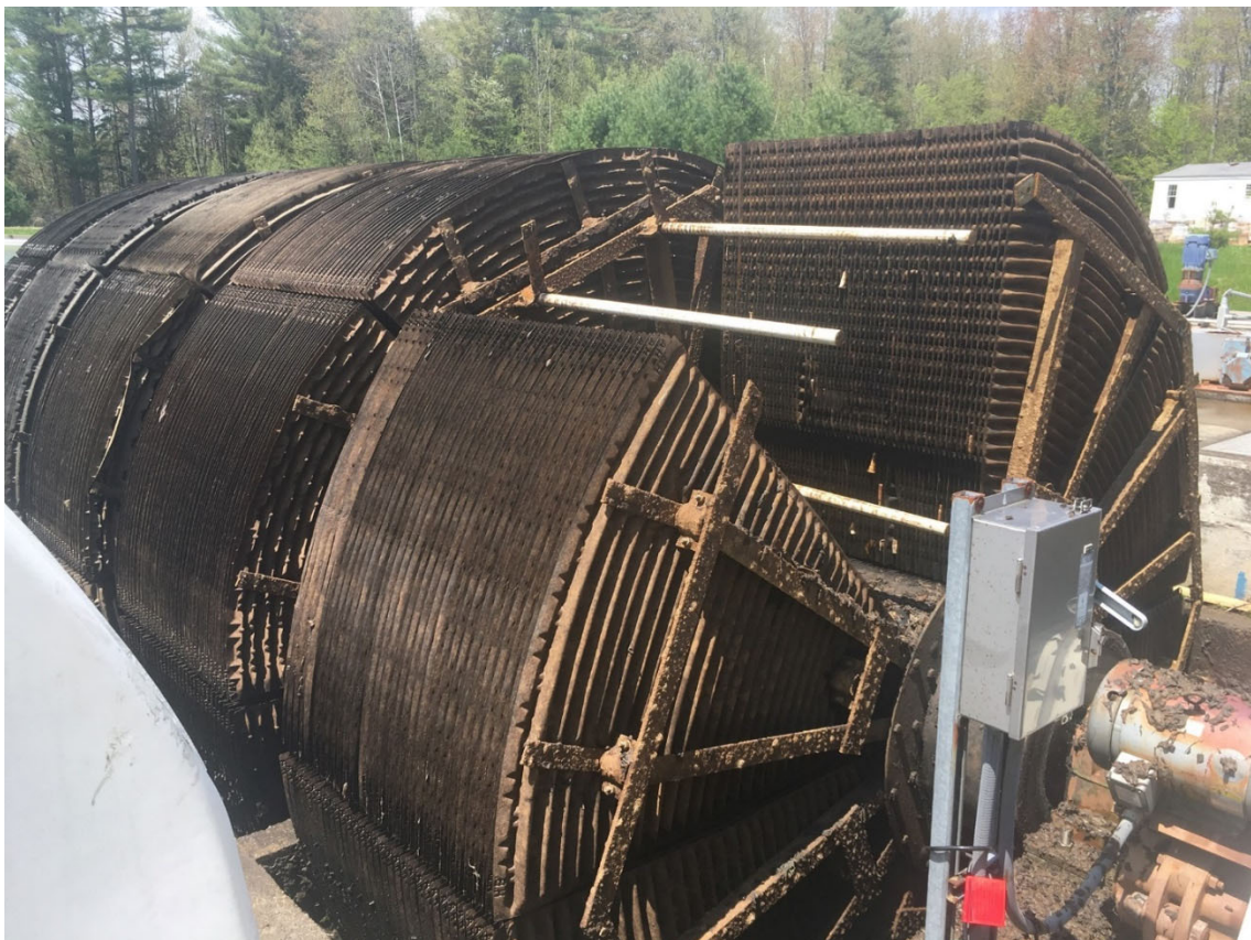
An RBC with one section removed.
