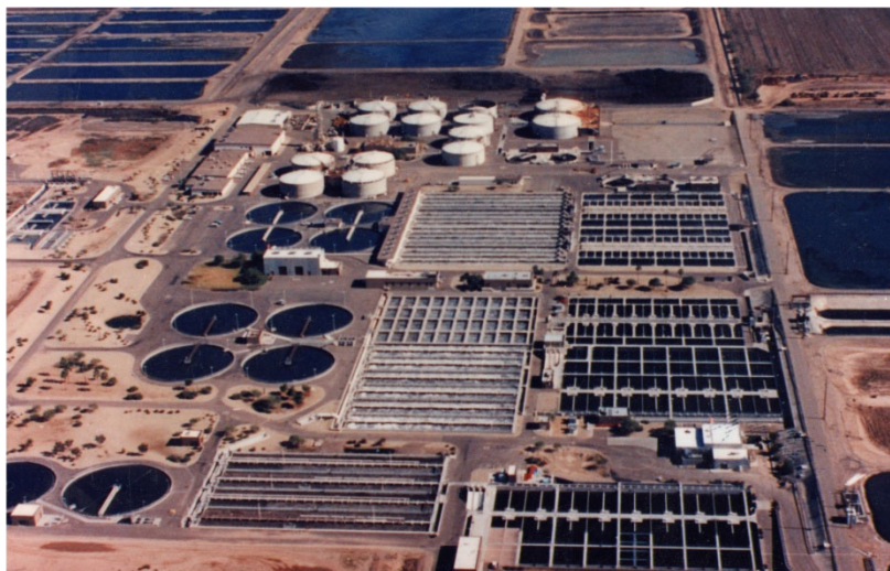
Modern wastewater treatment plant
