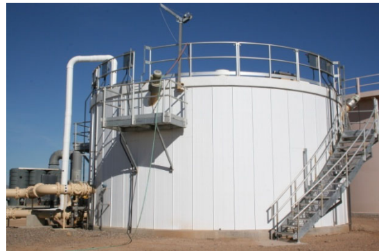
Anaerobic Digester
