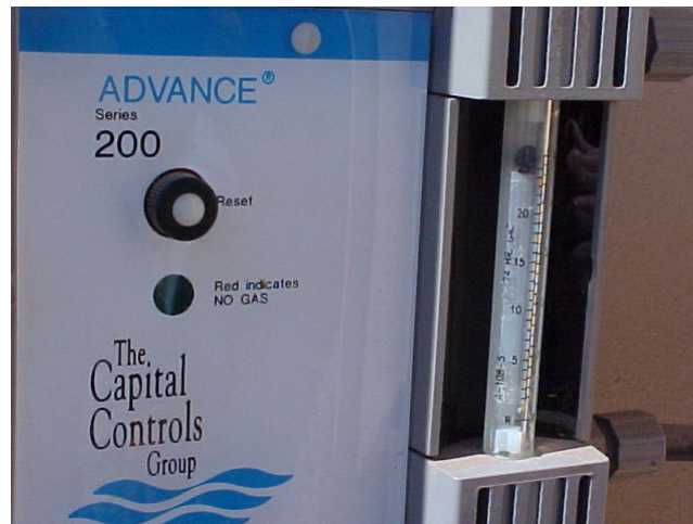
Chlorine measurement devices or Rotometers.
