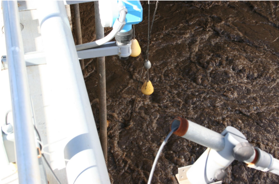
Old mixed liquor. The dark color is an indicator of old bugs or upset.
