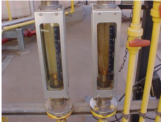
Chlorine measurement devices or Rotometers.
