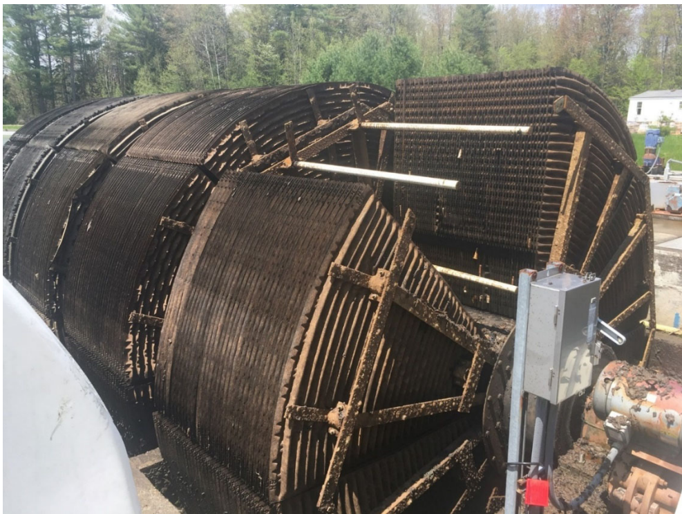
An RBC with one section removed.
