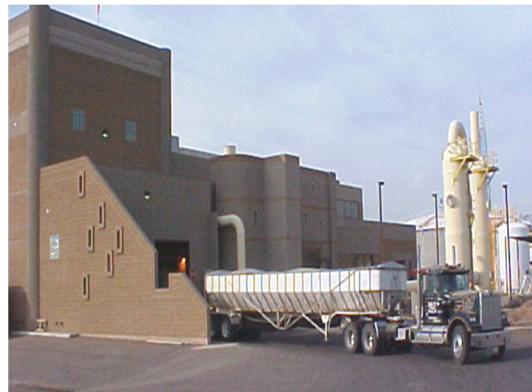
Large solids handling facility
