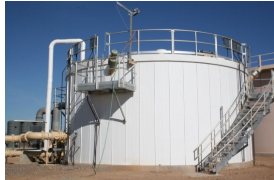
Anaerobic Digester
