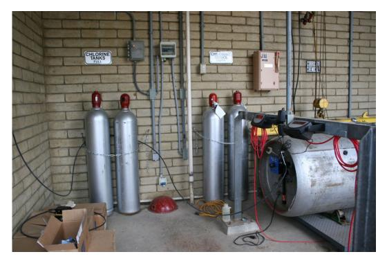
500-pound chlorine container and 150-pound chlorine gas cylinders. The 1/2 ton is on a scale. Cylinders stand upright and containers on their sides.
