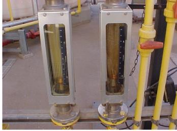
Various Chlorine measurement devices or Rotometers.
