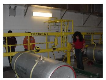
Chlorine leak detection equipment may not be required for very small chlorine rooms with an exterior door (i.e., floor area less than 3m<sup>2</sup>).
