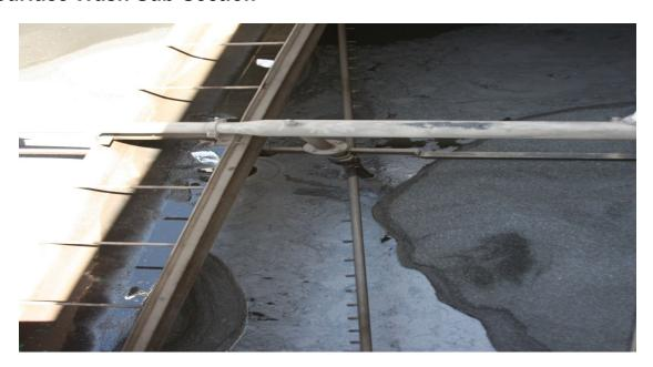
The photograph above shows a drained filter with the surface wash agitator and nozzles exposed. During operation these will spin, spraying water during the water backwash.
