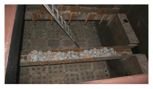
The photograph above shows a filter support bed under construction.
