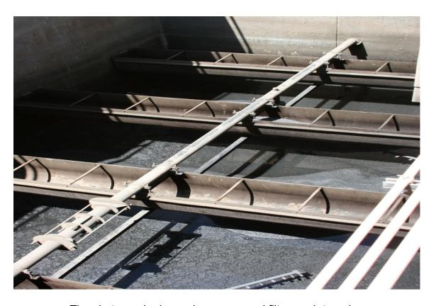
The photograph above shows exposed filter wash troughs.
