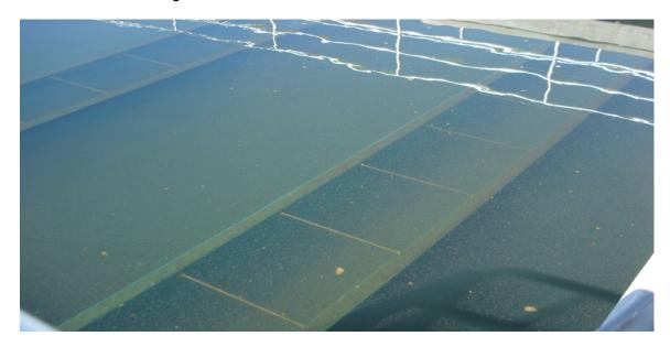
The above photograph is a filter from a direct filtration plant; notice the size of the floc – a good size for filtration.
