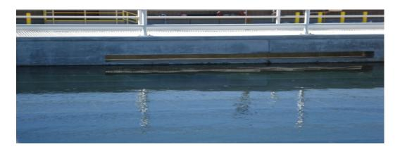
The photograph above shows the overflow wall opening in case the filter level gets too high.
