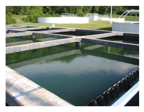
Top Photograph - Final Rectangular Sedimentation Basin Discharge Weirs
