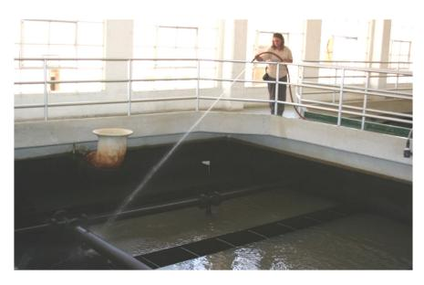
In the photograph above, overfeeding flocculants to meet federal regulations caused Iron to precipitate on the filter walls, resulting in this dark stain.
