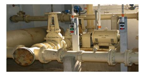
Both photos are of essential components of the backwash equipment for the water plant: an elevated storage tank and/or backwash pumps.
