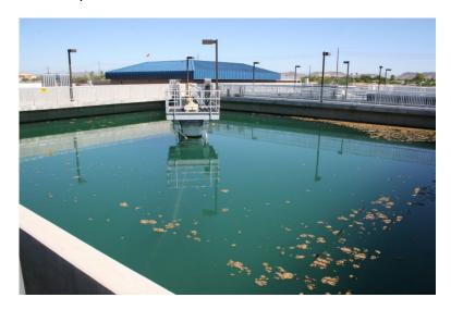
Let's first look at the components of a rectangular clarifier. Most are designed with scrapers on the bottom to move the settled sludge to one or more hoppers at the end of the tank. It could have a screw conveyor or traveling bridge used to collect the sludge. The most common is a chain and flight collector. Most designs will have baffles to prevent short circuiting and scum from entering the effluent.
