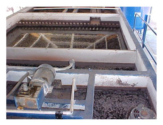
Example of a small water treatment package plant with coagulation, flocculation and filtration all within a 20-foot area.
