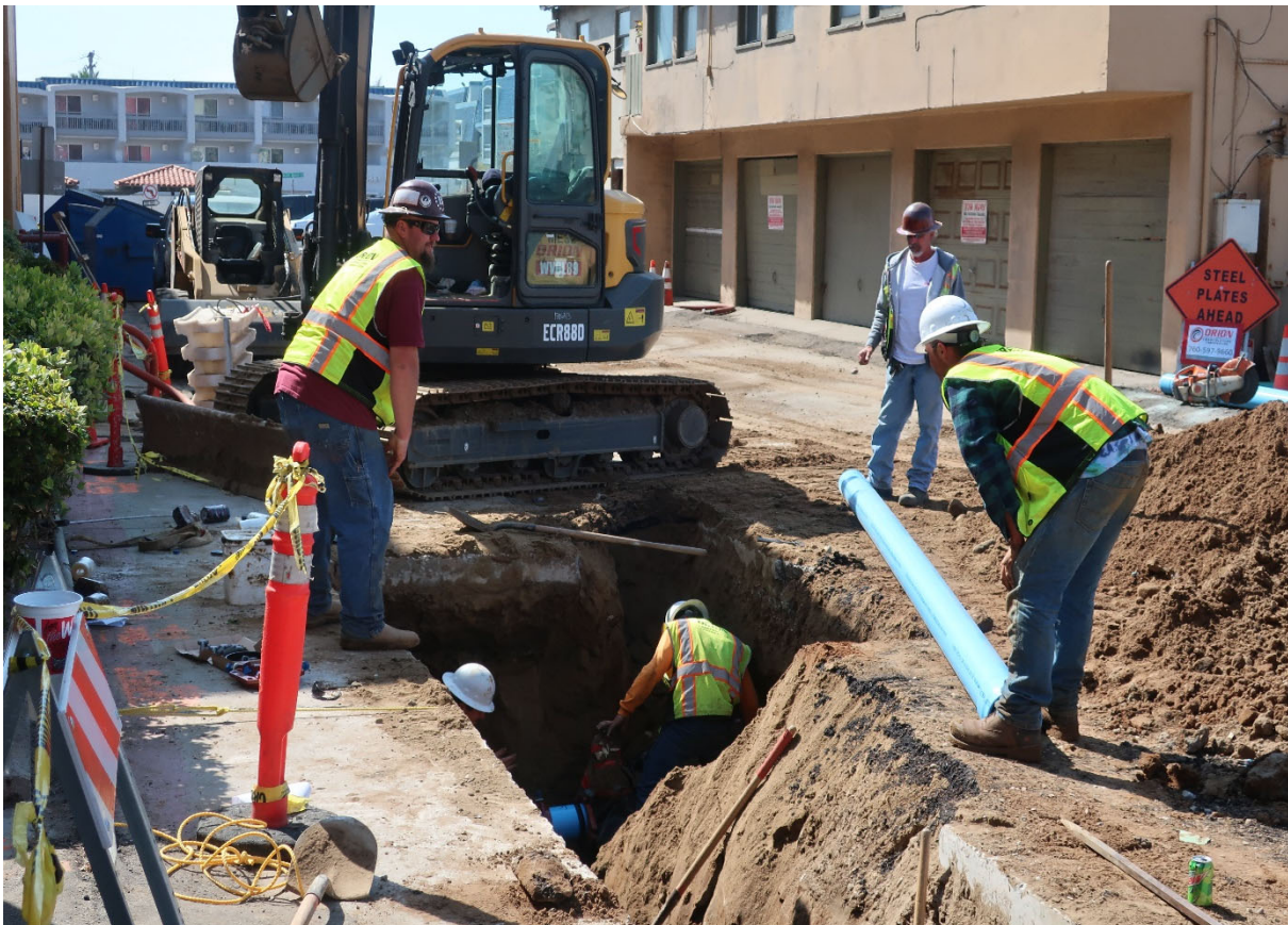
Replacing a section of plastic water main
