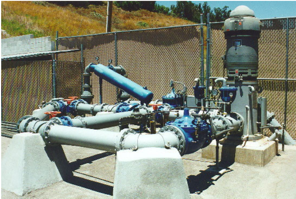
VERTICAL TURBINE WELL EXAMPLE
