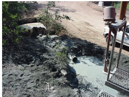
Constructed Mud Pits
