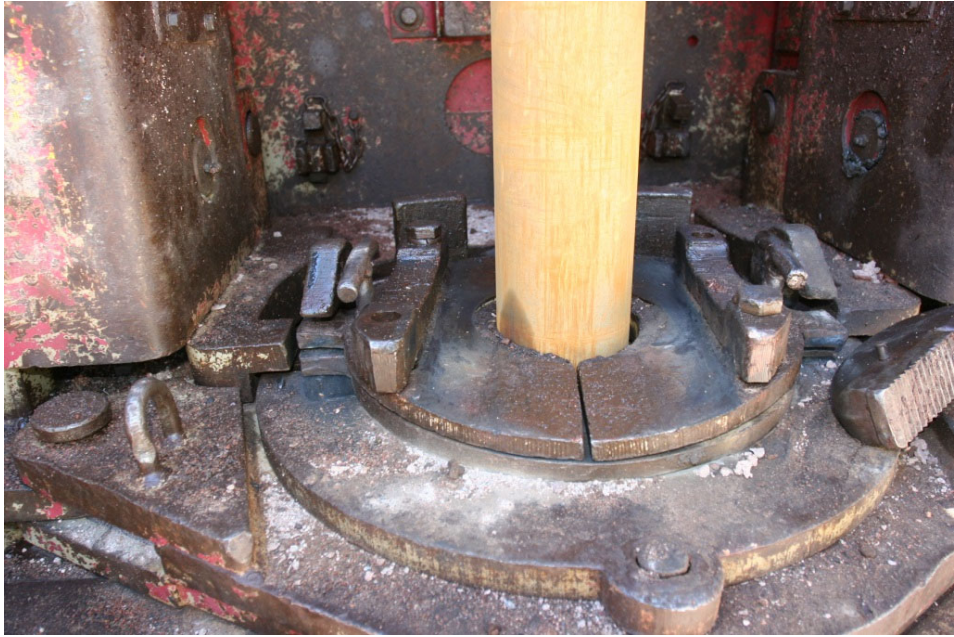
Top, drilling deck, below, well secured under drilling deck with pipe and pipe slip.
