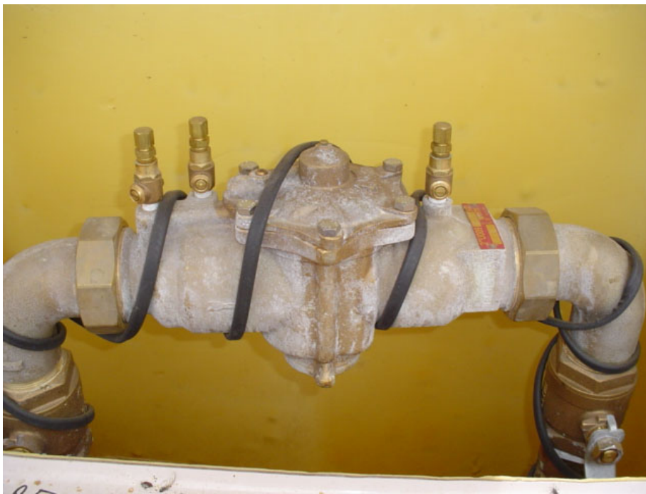
Top photo, a Hot Box, a good method of keeping the assembly from freezing during the winter. Bottom, electrical heat tape method for freeze protection.
