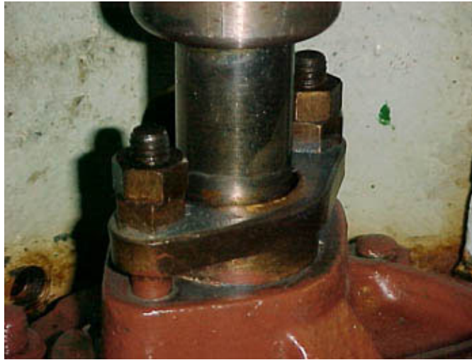
PUMP PACKING BOX WITH ADJUSTMENT LOCK NUTS
