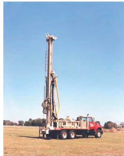
Typical Rotary Rig
