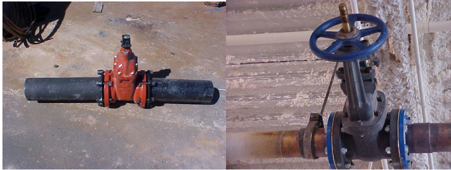
Different types of Gate Valves. (Linear)
