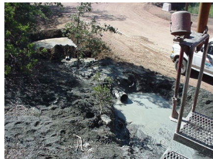
Constructed Mud Pits
