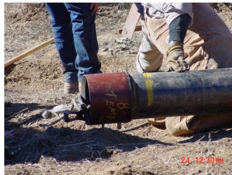
The Cutting Shoe is welded to the bottom of casing before installation.
