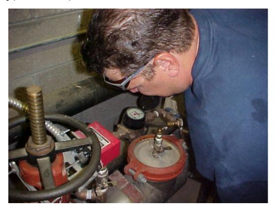
A Certified Backflow Tester (Jerry Durbin) examining a Double Check Detector check fire line assembly.
