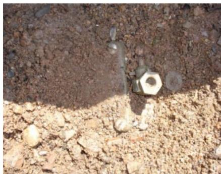
Another buried RP assembly deep inside a vault, all we can see is a test cock. All RPs need to be installed 12 inches above the ground. This device was buried in ground and not tested for over 25 years. Owners are required to test their devices once a year at a minimum.
