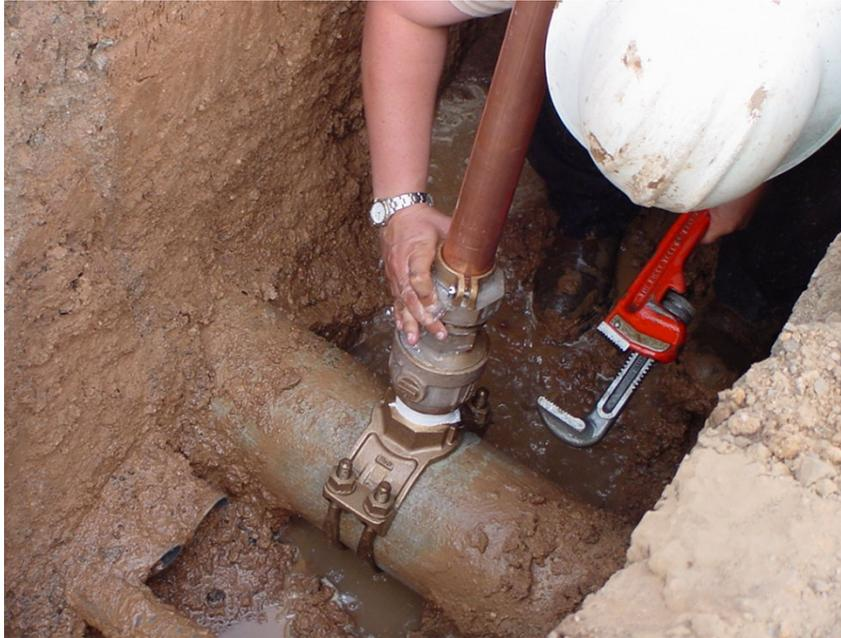
A water service worker installing a new copper water service line on an asbestos cement water main. Notice the bronze saddle with a corporation stop, a compression type fitting and a locking nut to secure the copper pipe to the corp. Bottom photo, the saw blade hole saw type tapping machine which was used to tap the main for the new service. This was completed with the water main under pressure so that other customers on the main did not have their water service disrupted due to the new service.
