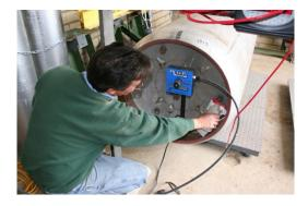
Here is an operator checking for Cl<sub>2</sub> leaks with Ammonia. If there is a Cl<sub>2</sub> leak, you will be able to see a white smoke. Even if you cannot smell the chlorine, the ammonia will find the leak.
