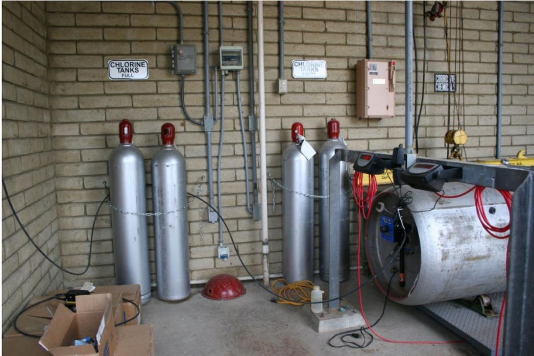
In the photo, we have a 1-ton chlorine gas container and 150-pound Cl<sub>2</sub> gas cylinders. The 1-ton is on a scale. Cylinders stand up-right and containers on their sides.
