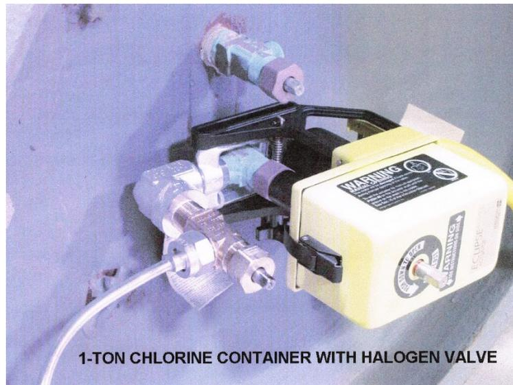
1-TON CHLORINE CONTAINER WITH HALOGEN VALVE
