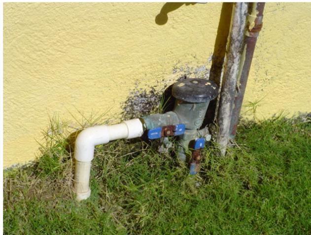
This PVB is not 12 inches above the ground nor the highest downstream outlet.
