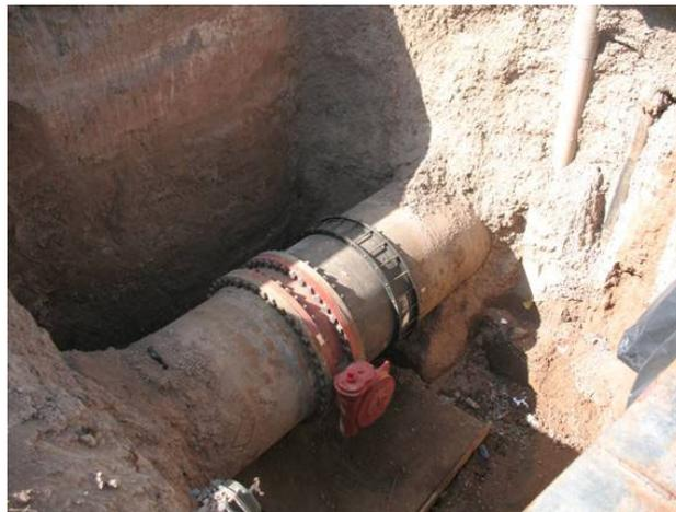
54-inch Butterfly valve on a huge transmission line. Nice job but no shoring, no ladder or valve blocking.
