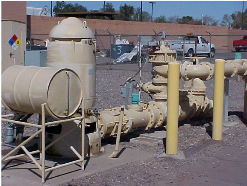
Well with a mineral oil sealed vertical turbine pump
