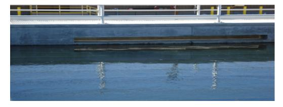
The photograph above shows the overflow wall opening in case the filter level gets too high.
