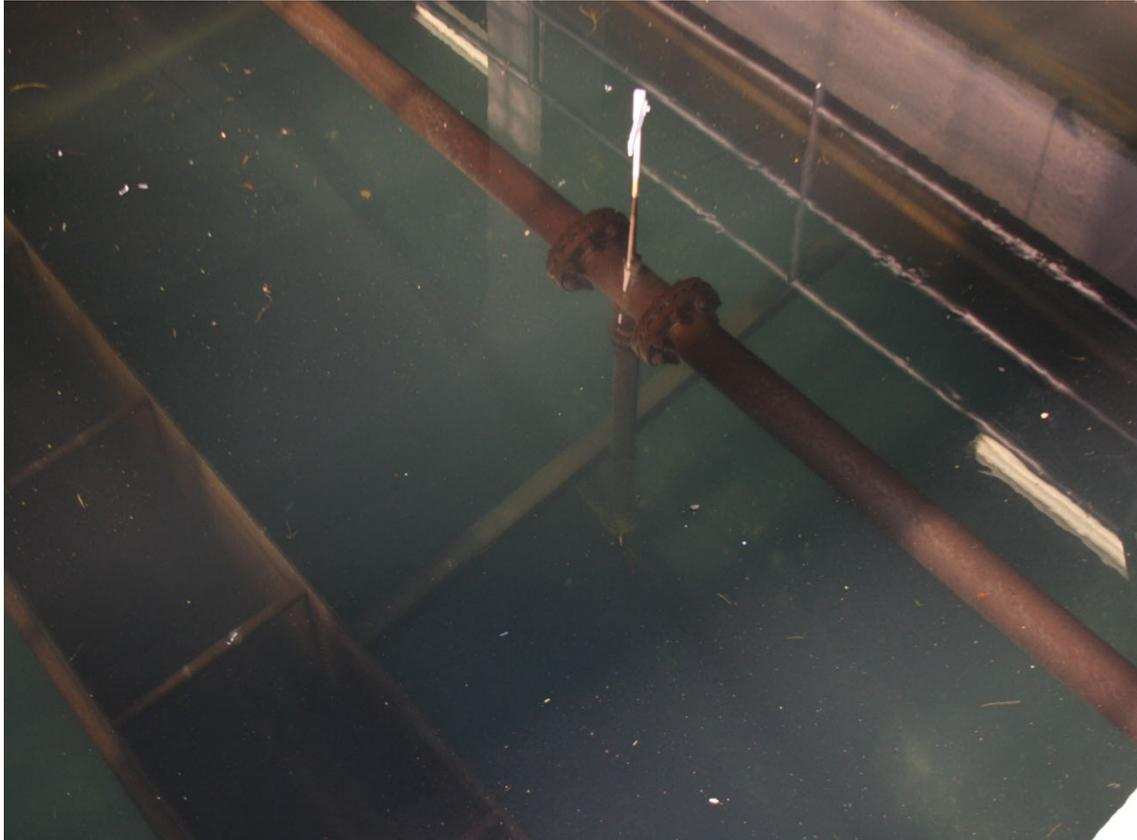
Mudballs can be seen on the top layer of the media bed or during the backwash water cycle. Typically, these will not flow over into the filter troughs. Mudballs must be removed manually, generally requiring extensive filter media reworking.
