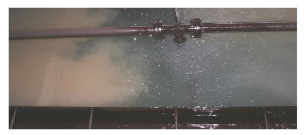
The surface wash system consists of a series of pipes installed in the filter that introduce high velocity water or air jet action into the upper layer of the filter. This jet action will generally be supplied by rotating arms that are activated during the backwashing of the filter.
