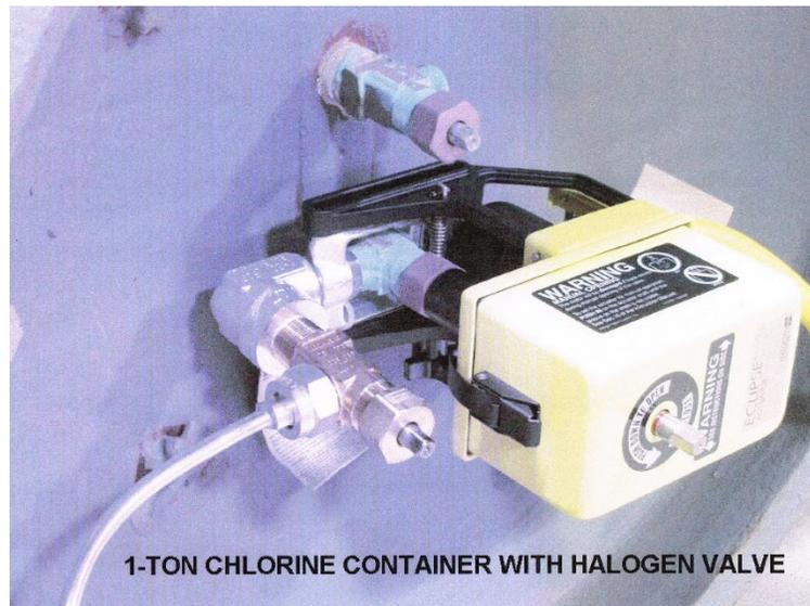
1-TON CHLORINE CONTAINER WITH HALOGEN VALVE
