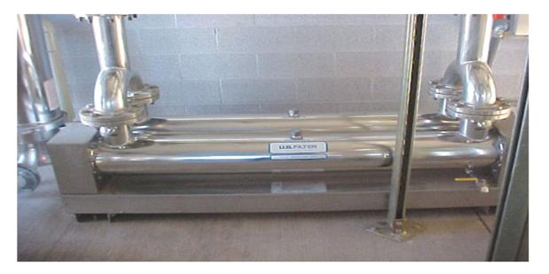
The lamp itself does not come into direct contact with the water, The lamp is placed inside a quartz tube, and the water is in contact with the outside of the quartz tube. Quartz is used in this case since practically none of the UV rays are absorbed by the quartz, allowing all of the rays to reach the water.
