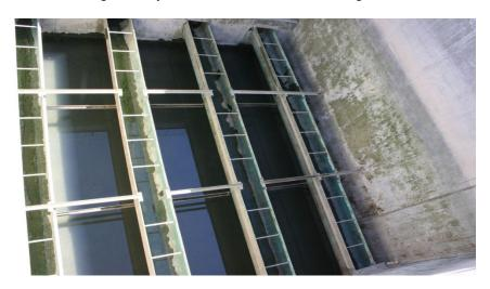
In this photograph, you can see the water lines on the wall of the filter. The deeper the water the more head pressure exerted on the filter media.
