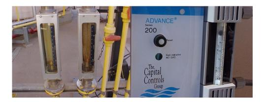
Chlorine measurement devices or Rotameters.
