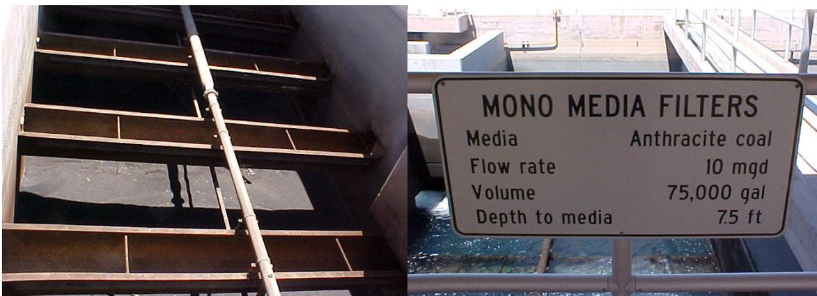
Dried backwash channels on the top of a cleaned filter bed.
