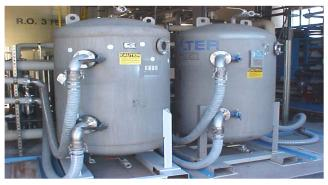
The use of two exchange materials makes it possible to remove both metal and acid ions from water. Some cities and towns, however, prohibit or restrict the use of ion exchange equipment on drinking water, pending the results of studies on how people are affected by the consumption of the added sodium in softened water. The commercial ion exchange containers hold the resin for the deionization.
