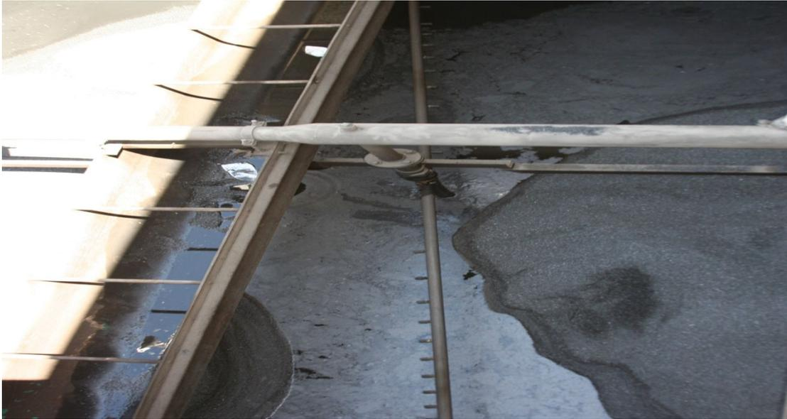
The photograph above shows a drained filter with the surface wash agitator and nozzles exposed. During operation these will spin, spraying water during the water backwash.
