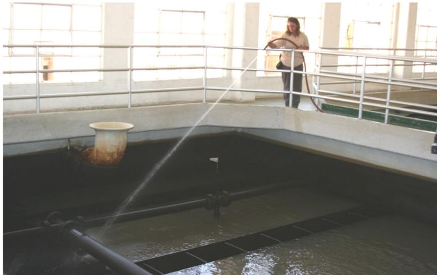
In the photograph above, overfeeding flocculants to meet federal regulations caused Iron to precipitate on the filter walls, resulting in this dark stain.
