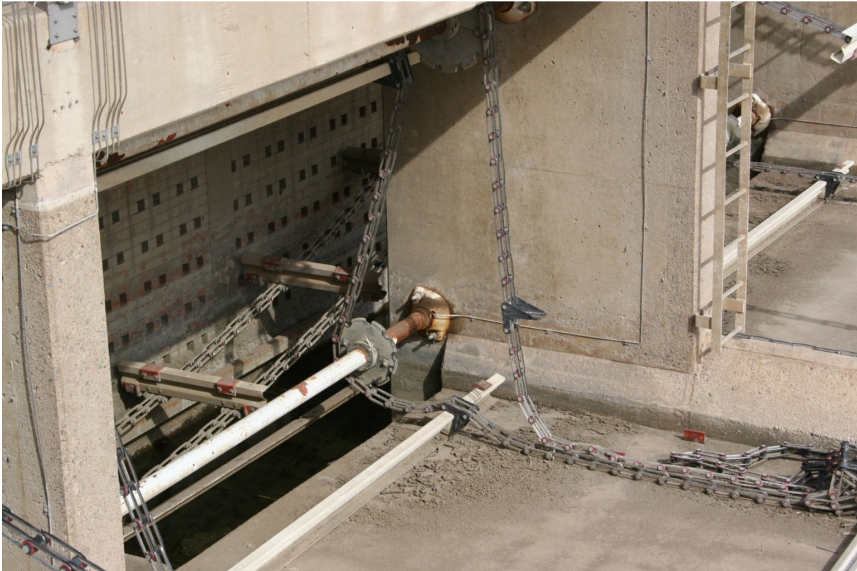
Rectangular basin flights and chains.
