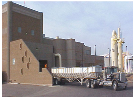
Large solids handling facility
