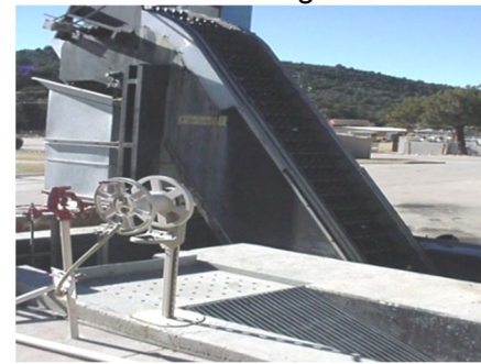
Manual and Mechanical Bar Screens
