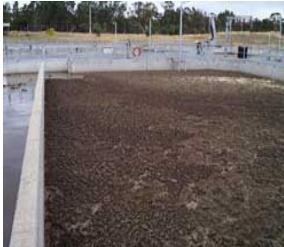
Figure 3. Dry Microthrix parvicella foam trapped in an anoxic zone of a BNR plant aeration basin.
