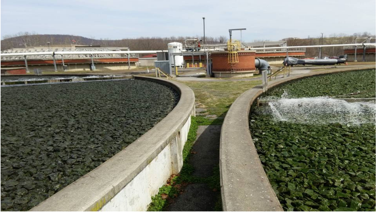
Fixed-film trickling filters. The left filter discoloration is due to sloughing. The photo below is the actual material off that filter.
