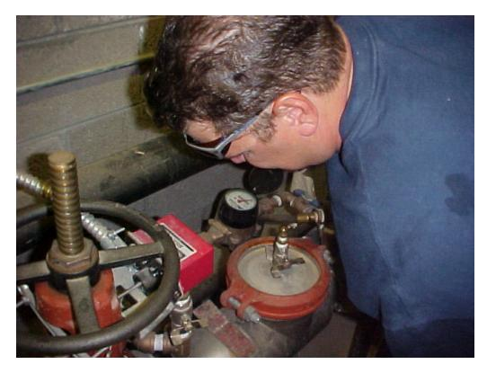
A Certified Tester is testing the integrity of this RP. Notice OS &Y.
