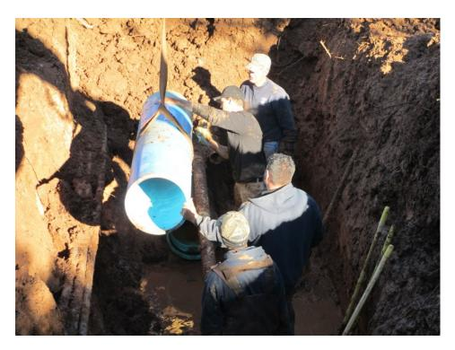
Wear appropriate personal protective equipment (PPE) as required by the task being performed and as required per OSHA regulations. Ensure a spotter is used if there are overhead power lines, underground utilities or tight working conditions in the work area. Verify the competent person is on site.
