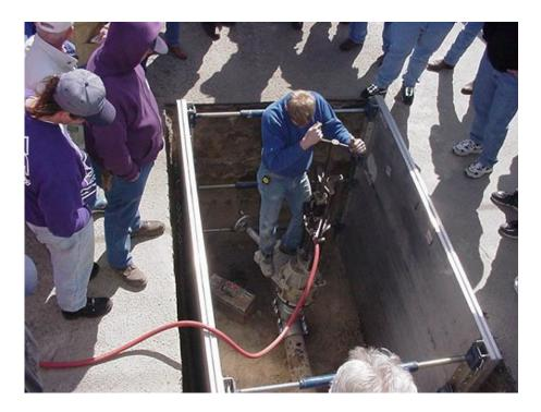
Hydro-Stop valve insertion machine
