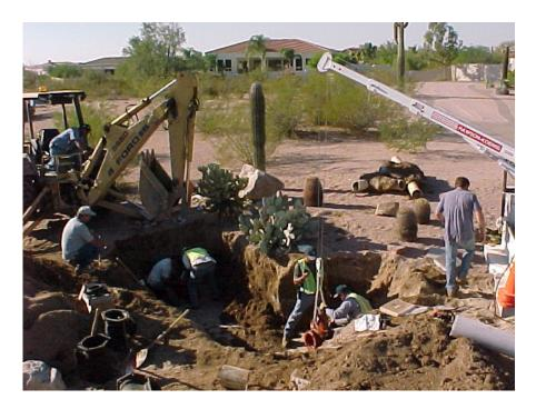
Top photograph, two gate valves blew out, you can see the kickers or thrust blocks remaining in the back ground. Bottom photograph, a tapping machine and a new gate valve. These tapping machines are very expensive.
