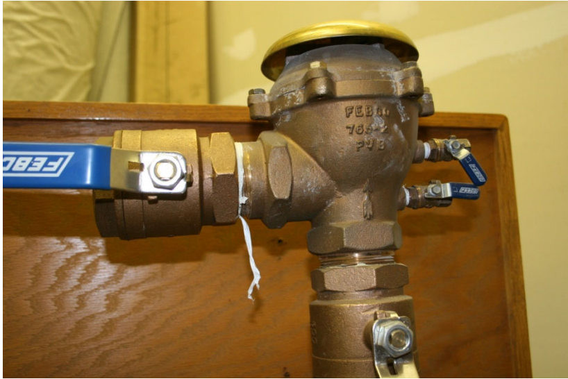
PRESSURE VACUUM BREAKER ASSEMBLY
