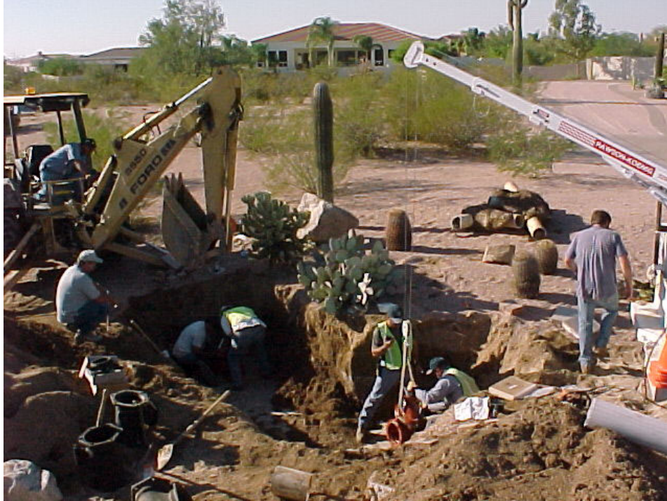
Top photograph, two gate valves blew out, you can see the kickers or thrust blocks remaining in the back ground. Bottom photograph, a tapping machine and a new gate valve. These tapping machines are very, very expensive.
