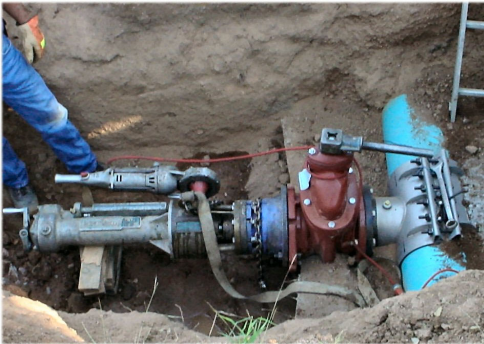
Top photograph, two gate valves blew out, you can see the kickers or thrust blocks remaining in the back ground. Bottom photograph, a tapping machine and a new gate valve. These tapping machines are very, very expensive.
