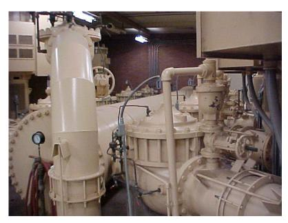
The inside of a booster pump station, notice the PRV with air relief valve.
