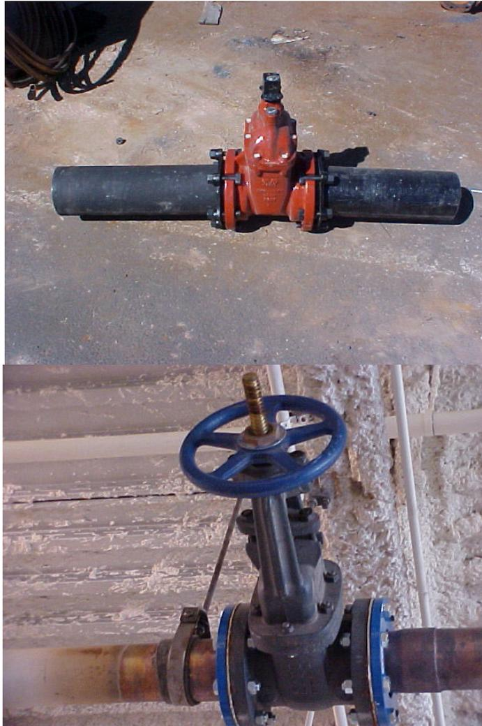
**Two different styles of Gate Valves.** Top photograph is valve ready for a valve replacement. Bottom photograph is OS&Y commonly found on fire lines. (Outside Screw and Yoke) As the gate is lifted or opened, the stem will rise.
