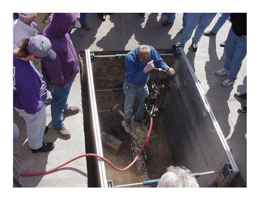
Hydro-stop valve insertion machine
