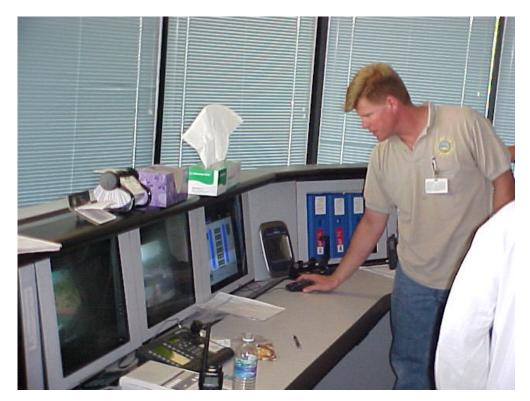
Here is an Operator who utilizes electronic or SCADA control of the valves at a modern treatment facility.
