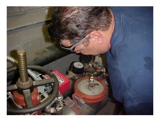
A Certified Tester is testing the integrity of this RP. Notice OS &Y.
