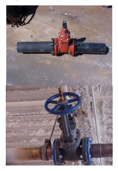
**Two different styles of Gate Valves.** Top photograph is valve ready for a valve replacement. Bottom photograph is OS&Y commonly found on fire lines. (Outside Screw and Yoke) As the gate is lifted or opened, the stem will rise.
