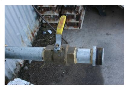
Most ball valves are the quick-acting type. They require only a 90-degree turn to either completely open or close the valve. However, many are operated by planetary gears. This type of gearing allows the use of a relatively small handwheel and operating force to operate a fairly large valve. Always follow standard safety procedures when working on a valve.
