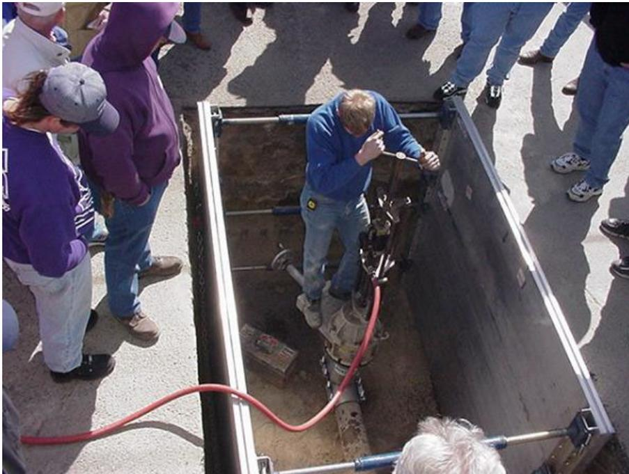
Hydro-stop valve insertion machine
