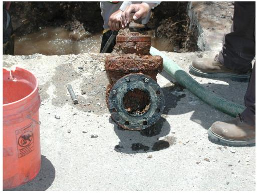
Here is a nasty 4 inch broken gate valve with serious Tuberculation. The valve is broken closed. The rust particles are sharp and can easily cut the water service worker. The flange bolts or Tee bolts were cut off to replace this valve. The rubber gasket will leave a black ink like stain on your clothes and in the water line as well. You will see lots of nasty stuff in the top portion of a valve. Some engineers or big shots refer to this area of the valve as the "Angular space".
