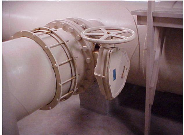
If the pipe is lined, make sure that the valve disc does not contact the pipe lining during the opening stroke. Contact with lining can damage the valve disc.
