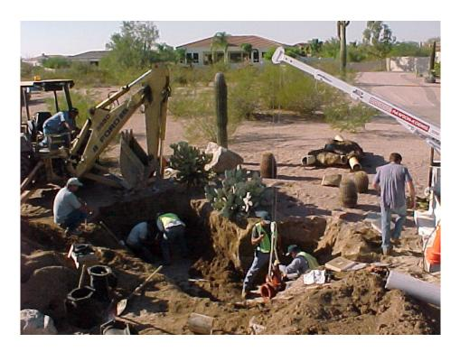
Top photograph, two gate valves blew out, you can see the kickers or thrust blocks in the back ground. Bottom photograph, a tapping machine and a new gate valve. These tapping machines are very, very expensive.
