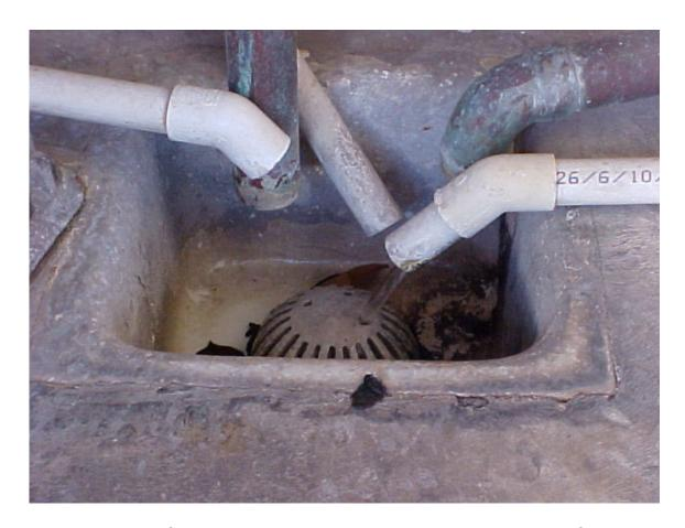
Which of these ice machine drains have an approved air gap?
