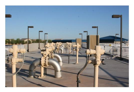
Here at a water treatment plant, we can see both valve actuators control devices and Butterfly valves as well. Bottom photograph is a cut-away of an actuator.
