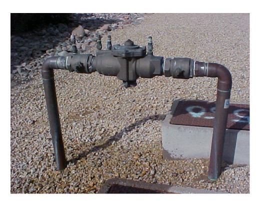
Leaky RP--have your assemblies tested annually or more often. Re-test after repairs and problems. A RP should not leak more that 1 or 2 minutes any more than that, there is a problem, a piece of debris or a stuck check is causing this RP's hydraulic relief port to dump.
