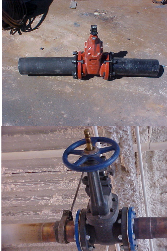
Different types of Gate Valves. (Linear)
