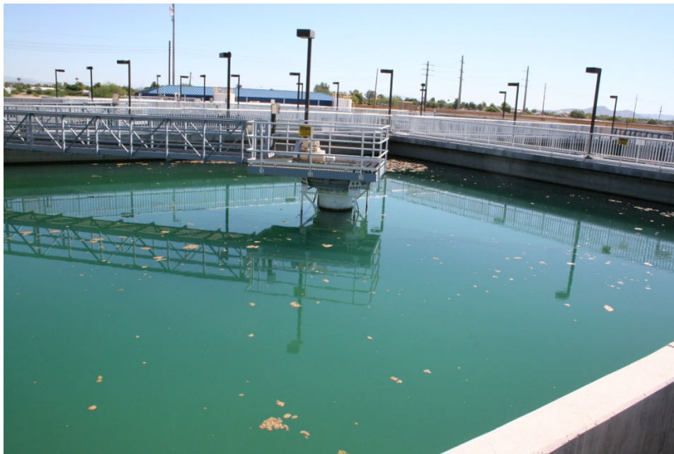
Top Photograph –Rectangular Clarifier
