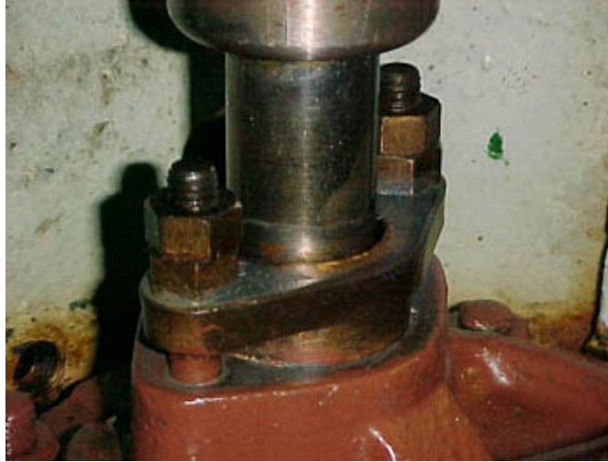
PUMP PACKING BOX WITH ADJUSTMENT LOCK NUTS
