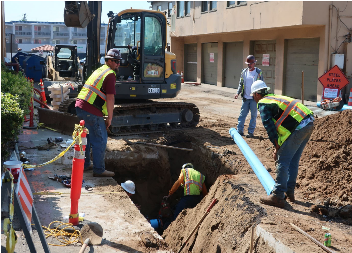
Replacing a section of plastic water main
