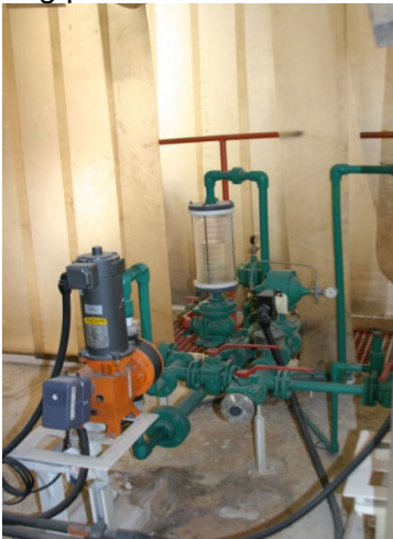
High rate feed pumps are used at this particular plant for Alum. The photograph on the right shows 3 positive displacement pumps in parallel operation.
