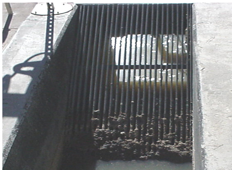
Mechanical bar screen, above photograph. Non-automated bar screen, below.
