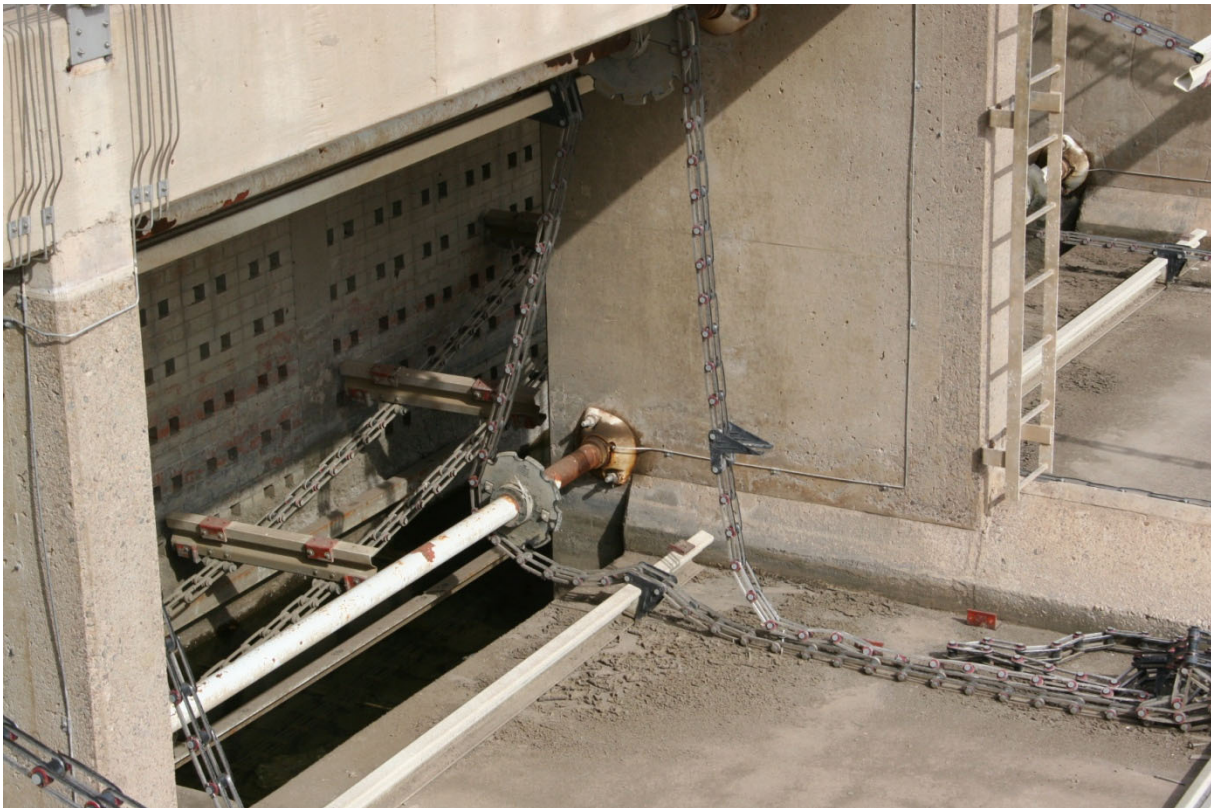
Rectangular basin flights and chains.
