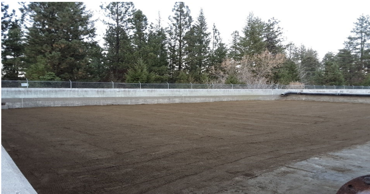
SLOW SAND FILTER These have become obsolete
