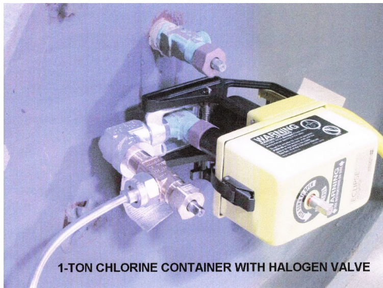
1-TON CHLORINE CONTAINER VALVES
