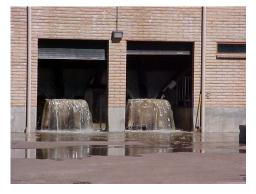
Domestic waste overflow at a WWTP headworks. Sometimes headworks do overflow, usually due to rags, grease and debris, or operator error. We do not like to see this happening!
