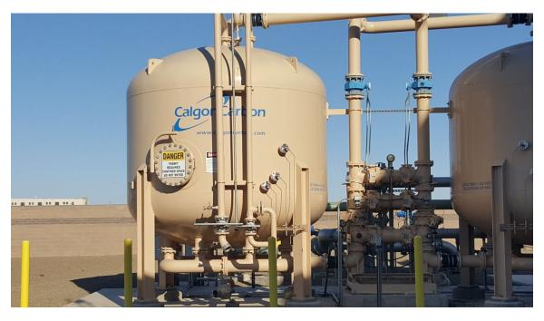
Granular Activated Carbon (GAC) vessel
