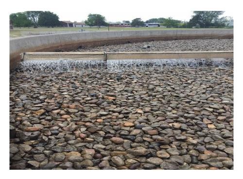
A TF consists of permeable medium made of a bed of rock (As seen above), slag, or plastic over which wastewater is distributed through the armature to trickle.
