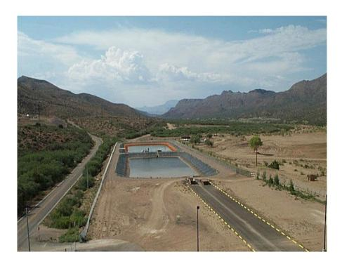
Lagoons in series. Some will argue that lagoons are not part an A/S process, but according the EPA, if you maintain suspended bugs for a process, it an A/S process.
