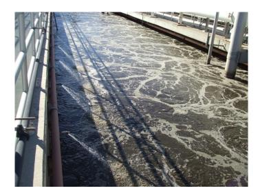
An activated sludge example of an aeration train or channel containing **m**ixed liquor (MLSS) in secondary treatment.
