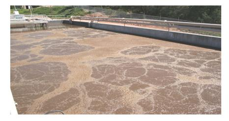
The above photograph shows air being unevenly distributed in an aeration tank.
