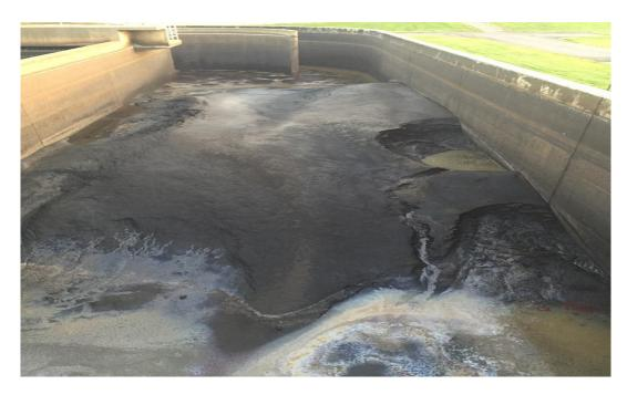
The results of not having grit removal. Filling part of an oxidation ditch aeration tank.
