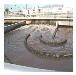
Oxidation ditch baffles slowing down the flow.
