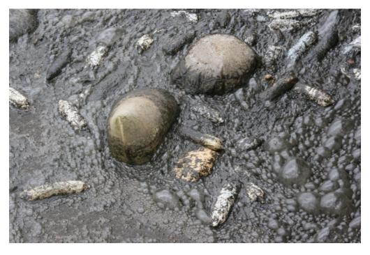
Floating scum in an influent chamber. This debris should be removed and sent to a landfill.
