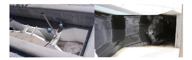
Sonic head (level) detection in the flume is used for flow measurement. Flow rates can be and used for flow weighted composite samples. Another application using sonic head level detection are weir boxes. Often referred to as a splitter box as illustrated below.
