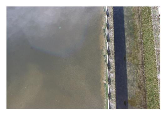
**Pin floc** being carried over the secondary clarifier weir due to a process upset. Ideally, the secondary effluent will be very clear. Excessive algae growth will create several different problems.
