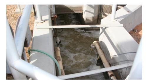
Aeration is often used to oxygenate the wastewater flow at the influent channel. **EXAMPLE OF FACT SHEET**
