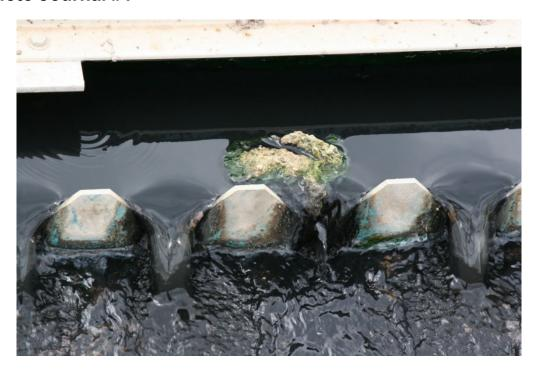
Caked grease (scum) stuck on a primary clarifier weir. Scum is normally scraped off and not sent to the downstream aeration tank.
