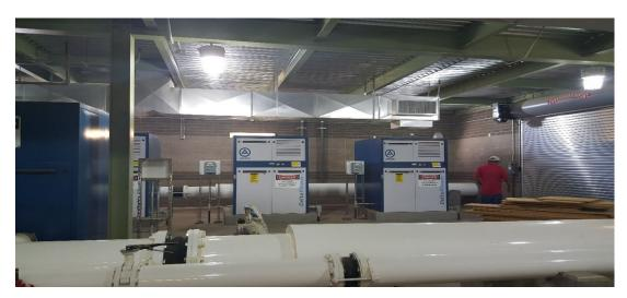
The above photo shows pipes and enclosed blowers as part of the aeration system. These areas are generally underground or in large buildings.
