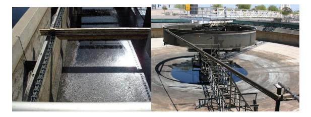
The photograph the left is a rectangular basin and on the right is a circular clarifier. The rectangular basin has chains and flights to scrap sludge and a circular basins use a slowly rotating raking mechanism.
