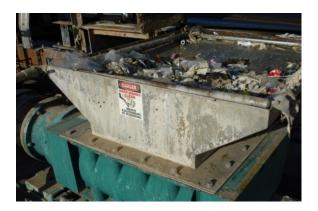
Grinder Pump: installed after the bar screens. The debris is sent to the landfill.
