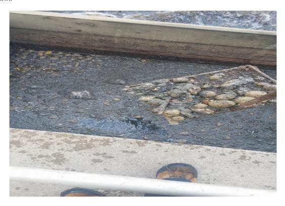
A buildup of grease balls in an oxidation ditch.
