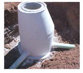
Grout is used to seal joints and prevent infiltration (I&I) into manholes or exfiltration out of the pipe.
