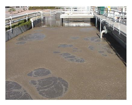
Activated Sludge Aeration Basin, identified by the bubbles.
