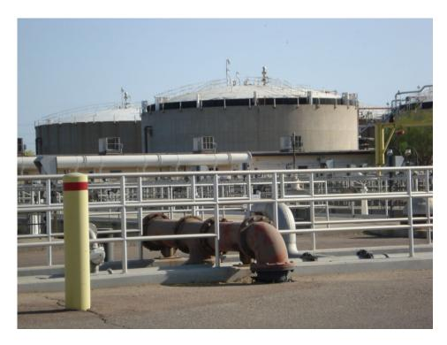
These two above ground circular tanks are massive anaerobic digesters.
