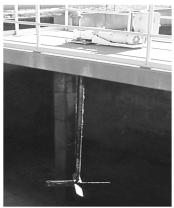
Other systems use both compressed air and a mechanical device to trap the bubbles. In one such system, submerged turbine aeration, air is injected below a rotating turbine blade that shears and disperses the air. Submerged turbine applications have also used a draft tube operating in a downdraft-pumping mode.
