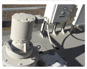
For the motor on this fixed bridge, aeration motor speeds are usually in the 1,800 rpm range. This speed is reduced to the 30 to 70 rpm range with gear reducers.
