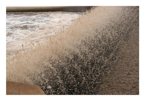
The rotor used above is for increase oxygen and mixing in an oxidation ditch.
