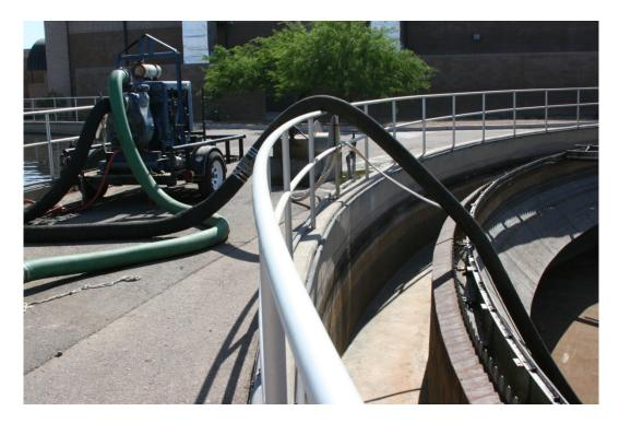
This circular clarifier has been dewatered with a portable pump Maintenance on a circular clarifier should be performed annually.
