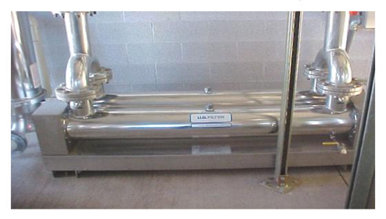
Enclosed lamp system, this one is on wastewater effluent.
