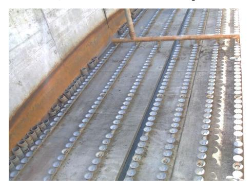
Porous air diffusers in an aeration tank.
