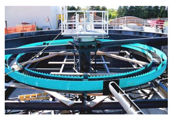
Holes in the bottom of the channel allow the influent to flow into the clarifier. The channel helps distribute the influent flow over the clarifier surface. Peripheral feed clarifiers may have either center take-off or peripheral.
