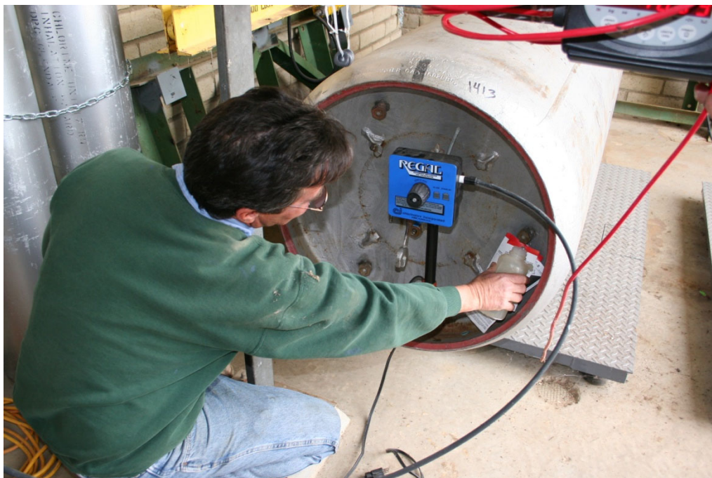
Top photograph, this blue device prevents the liquid from being pulled and freezing the lines. Bottom photograph, the application of an ammonia mist to detect a chlorine gas leak.
