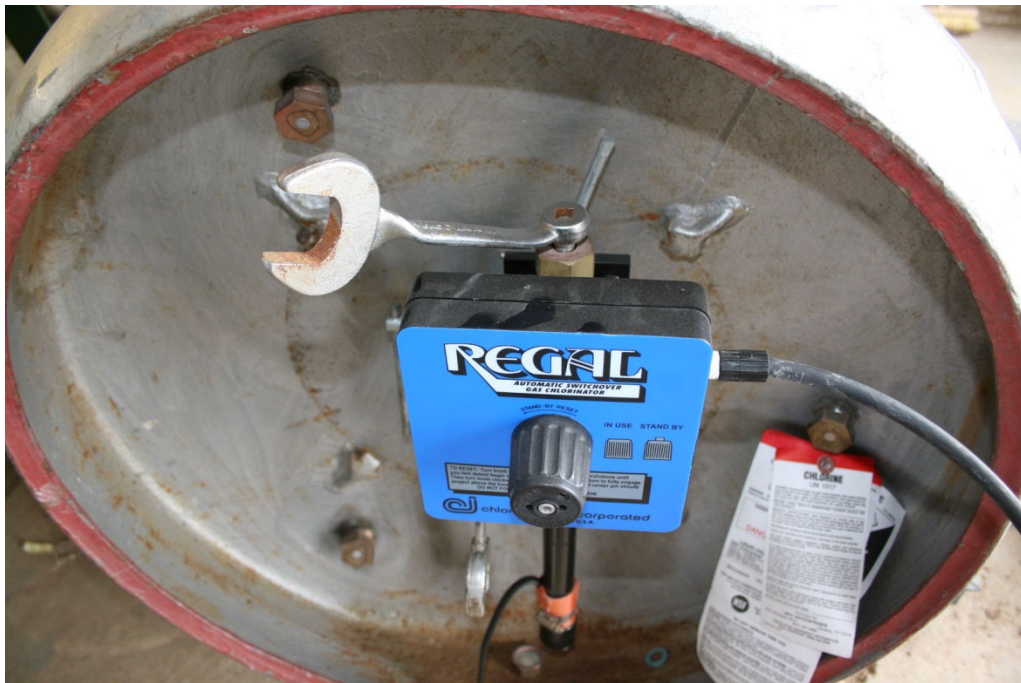
Top photograph, this blue device prevents the liquid from being pulled and freezing the lines. Bottom photograph, the application of an ammonia mist to detect a chlorine gas leak.
