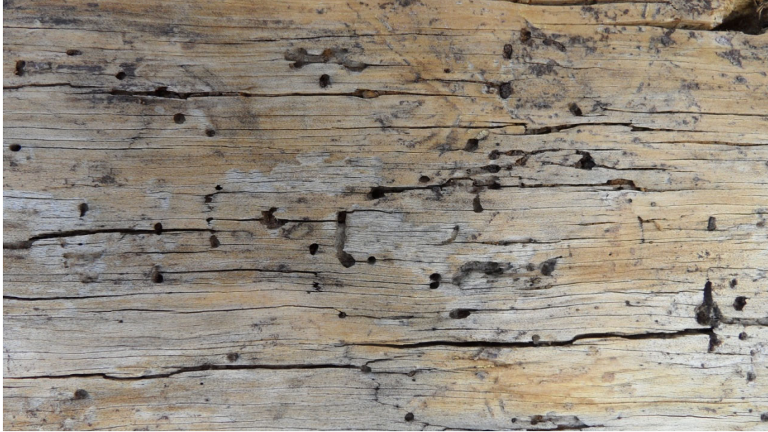
Evidence of Powder post beetles in above photo.
