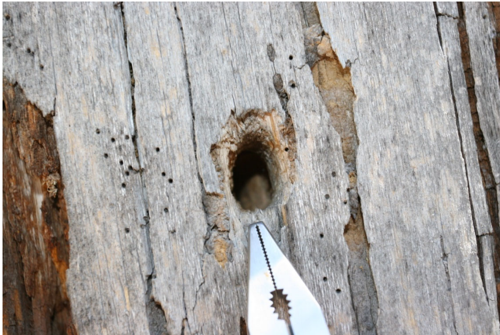
Evidence of Carpenter bee in above photo. Note Woodpeckers do not drill holes longer than their beaks. Woodpeckers are great wood destroyers, even on the sides of houses but the damage is only about 1 inch deep. You will probably go to prison if you try to control a woodpecker. Endangered species act and wildlife regulations are very strict.
