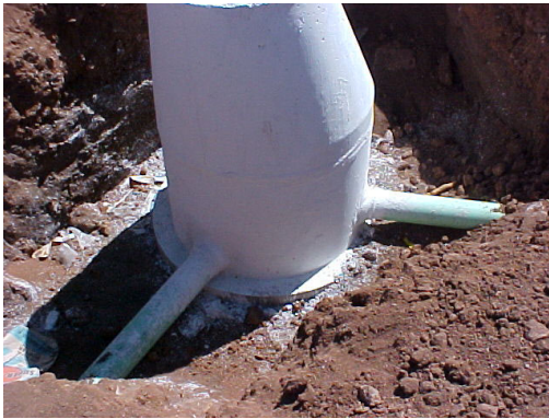
New sewer manhole with sewer mains before final burial.
