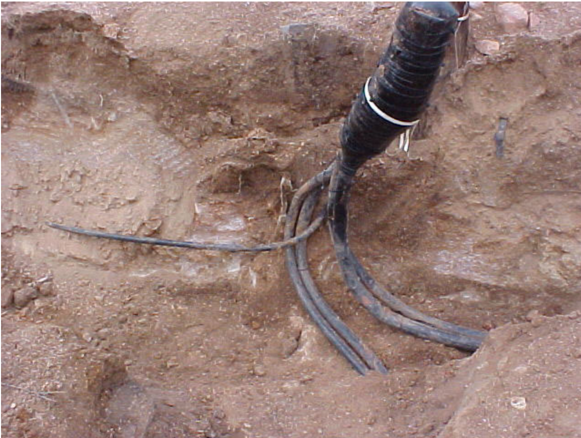
Telephone Cables, difficult to dig around, almost as digging near electric lines.
