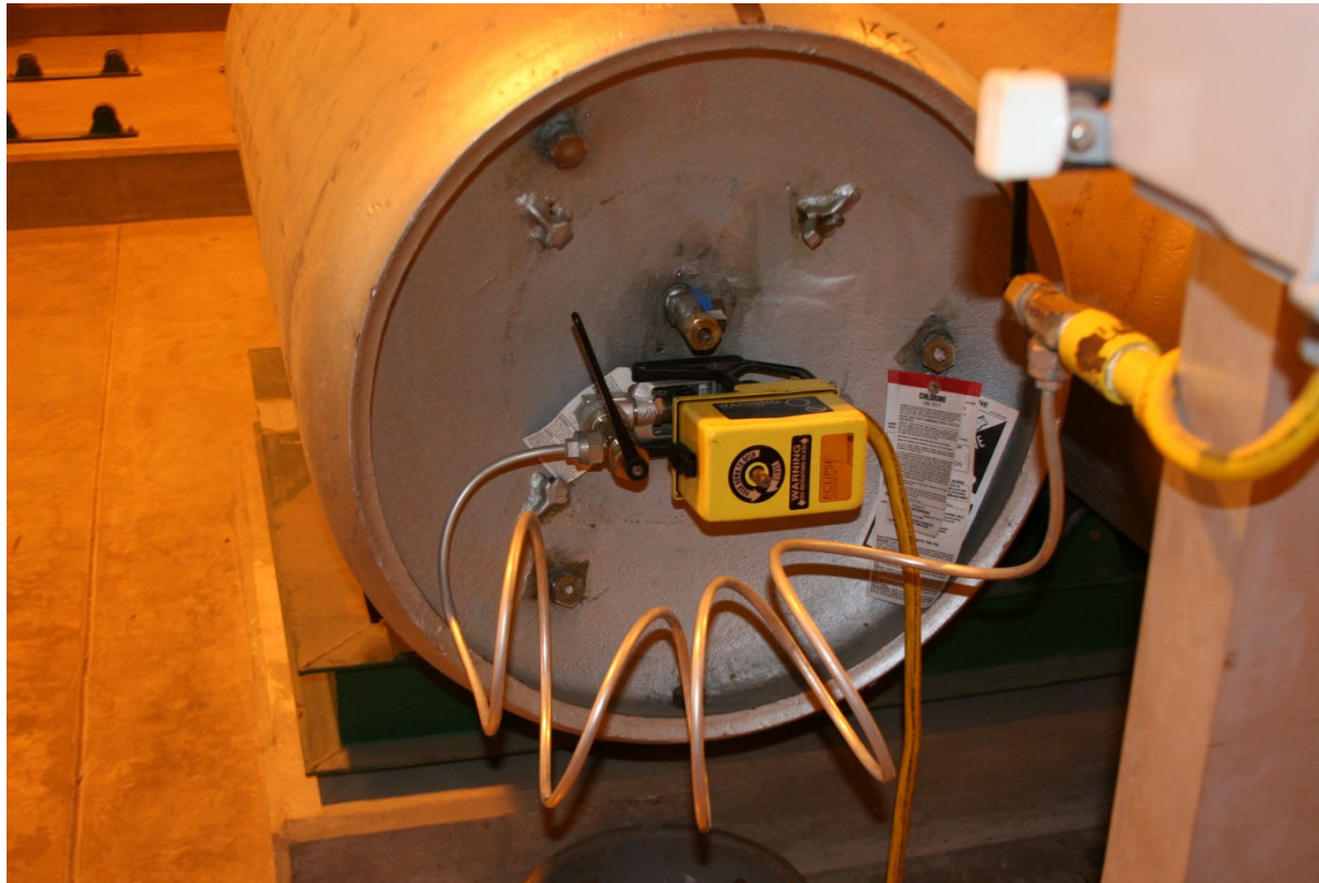
A 1-ton chlorine container.
