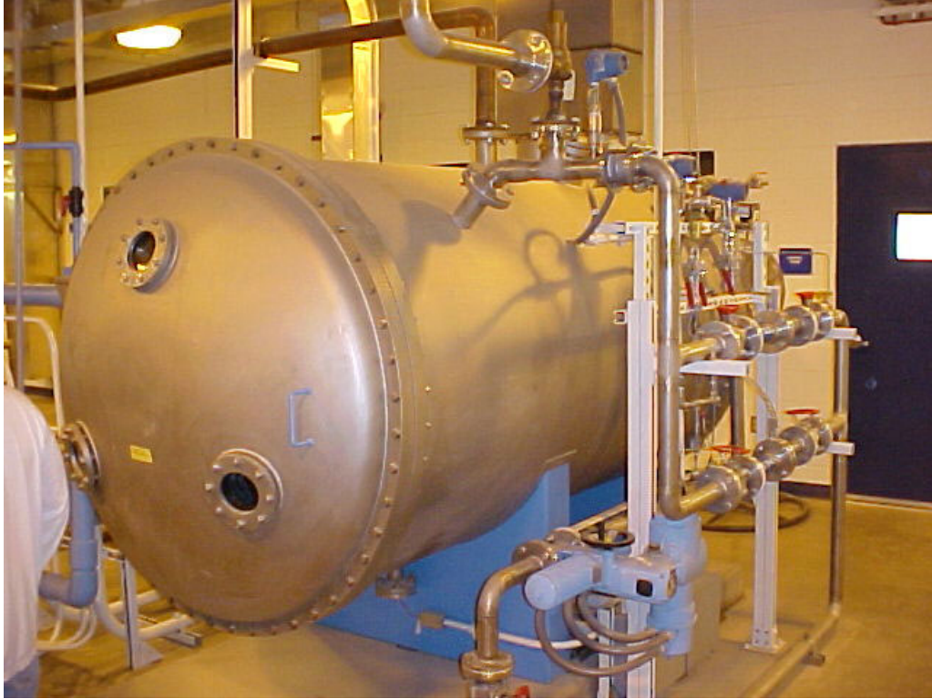
Ozone generator and control panel.
