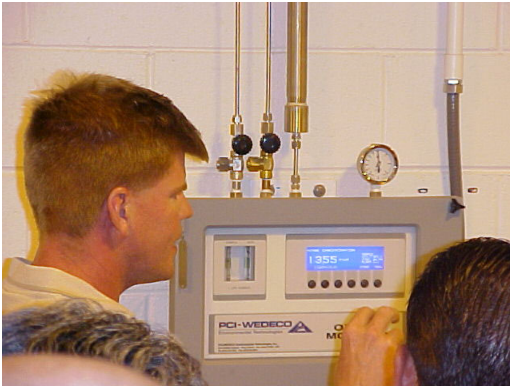
Ozone generator and control panel.
