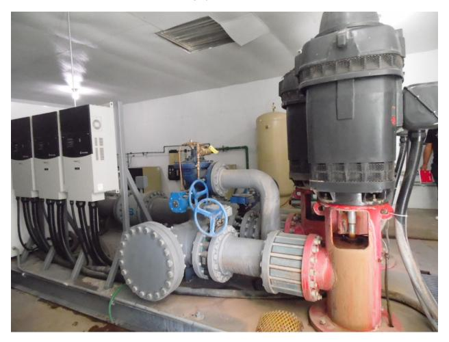
An **electric motor** is an electrical machine that converts electrical energy into mechanical energy. Most electric motors operate through the interaction between the motor's magnetic field and electric current in a wire winding to generate force in the form of rotation of a shaft.
