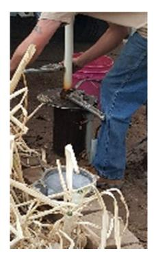
Attachment that screws into well pipe to be pulled. Metal disk supports couplings on wellhead while being pulled.
