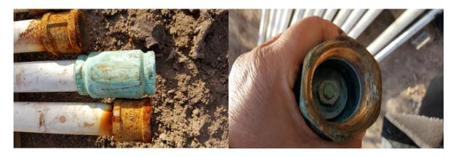
It is recommended to install a check valve every 100 feet of piping. Sometimes the valve becomes defective and causes pumping issues. When installing the the check valve, the correct direction of the check valve is important.
