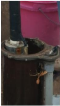
This pump has 16 stages and a 4 inch impeller. Rule of thumb, if you take the diameter of the impeller squared ( $4 \times 4$ ) and times it by the stages you will get the lift in feet. For example  $4 \times 4 \times 16 = 256$  ft of lift.
