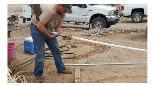
Each pipe section is 20 feet long. Here the attachment that screws into the pipe is being disconnected from the well rig.
