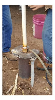
The wire gauge used is determined by volts, amps and the run. Care is taken not to tangle the wire while pulling the well and re-installing.
