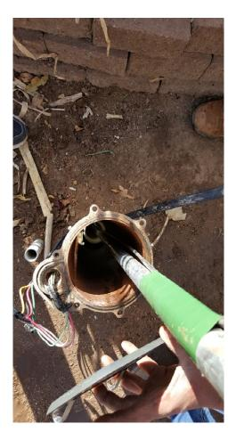
The discharge side of the pipe has a tee that seats on a saddle down below ground to prevent freezing.
