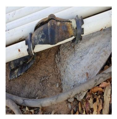
The submersible pump is about to be pulled out. Above, is the discharge side of the pump.
