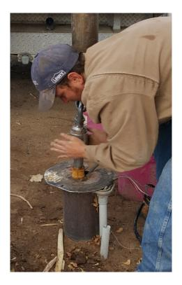
While pulling the PVC, care is taken not to damage electrical wiring. Next to the casing is conduit that runs from the electrical panel to the well.
