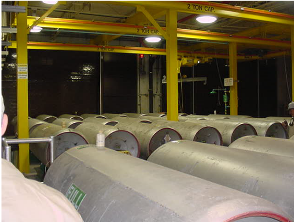
1-ton chlorine gas containers
