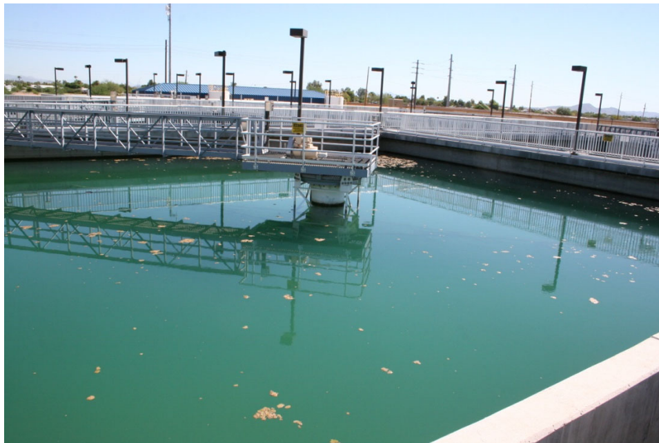
Top Photograph –Rectangular Clarifier
