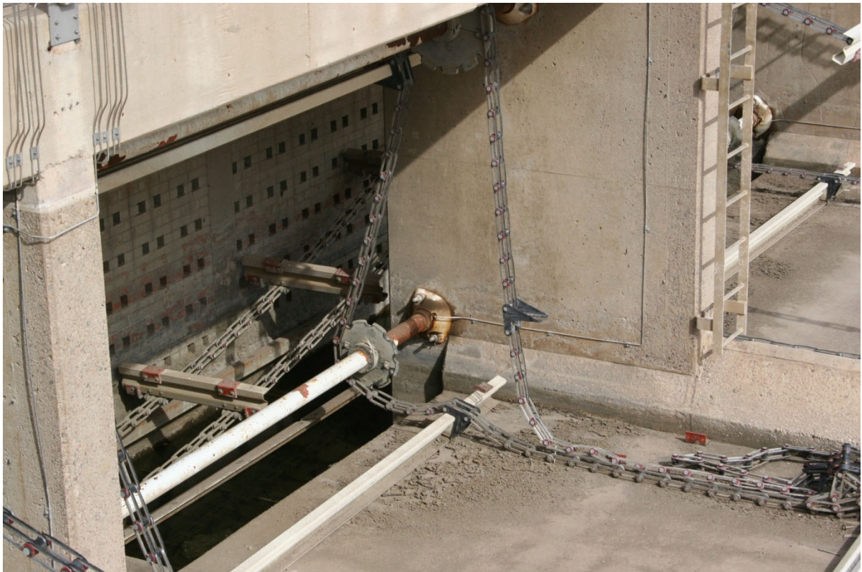
Rectangular basin flights and chains.
