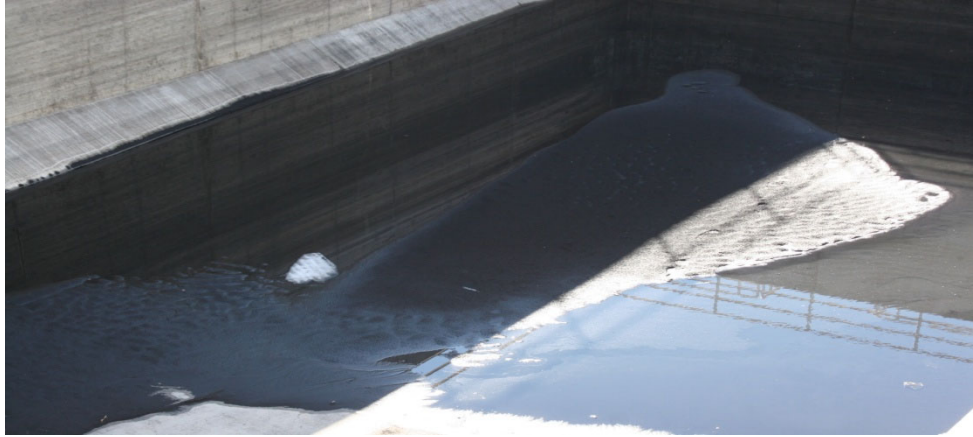
A backwash basin that has wasted or lost media caked on the bottom.
