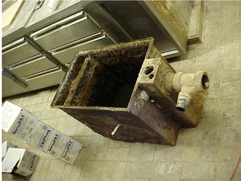
Infloor grease trap being removed and replaced with a grease interceptor.
