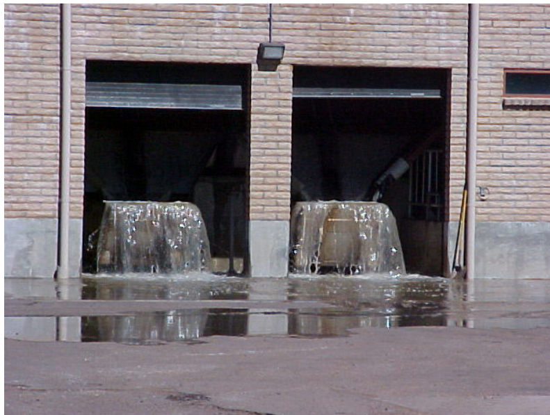
Headworks overflowing due to a blockage.
