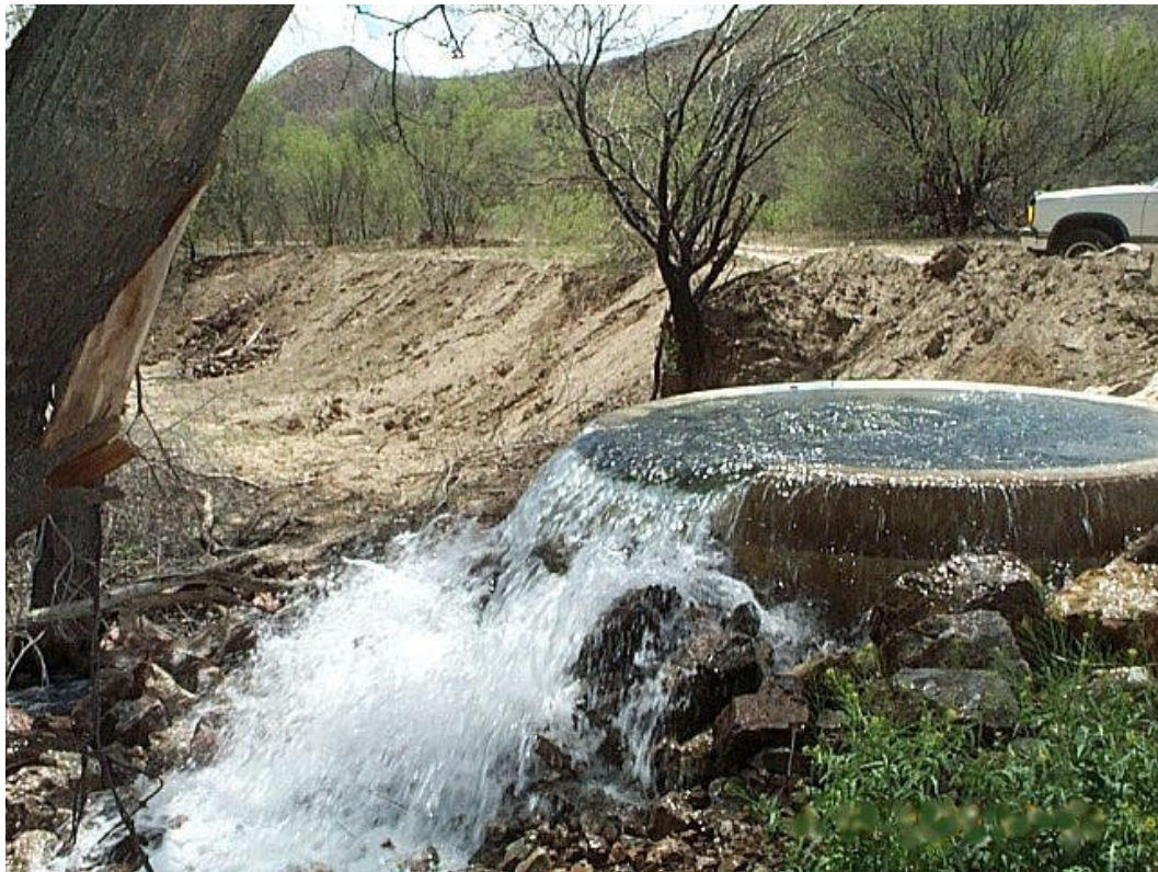
Treated wastewater outfall.
