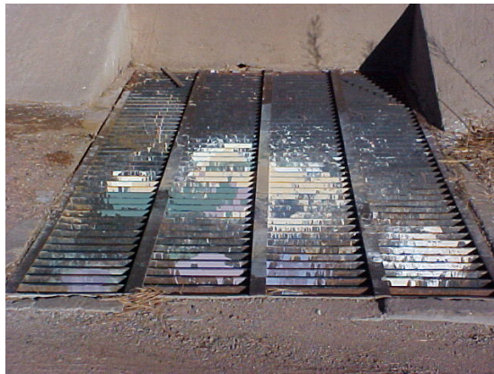
Evidence of illegal paint and chemical dumping.
