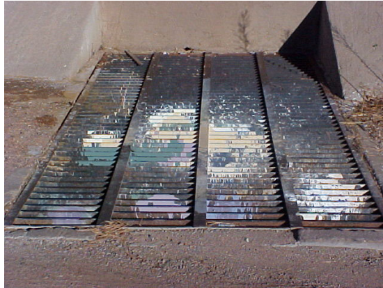
Evidence of illegal paint and chemical dumping.
