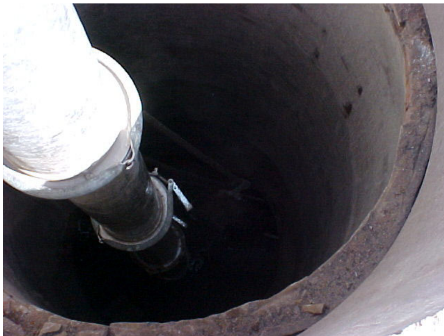
A Vector clearing a Manhole.
