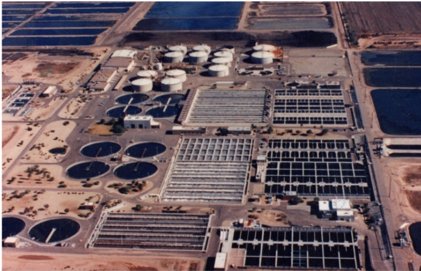
Large wastewater treatment plant
