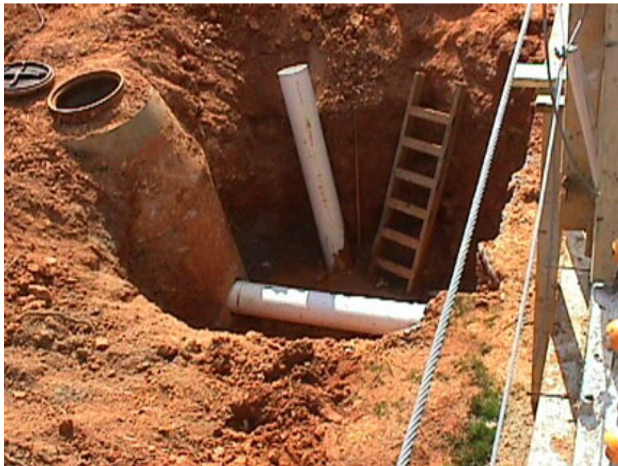
Sewer lateral going into a manhole.
