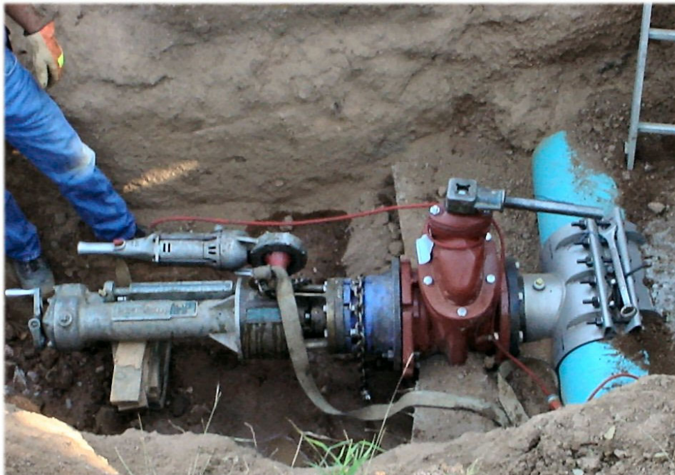
Top photograph, two gate valves blew out, you can see the kickers or thrust blocks in the back ground. Bottom photograph, a tapping machine and a new gate valve. These tapping machines are very expensive.
