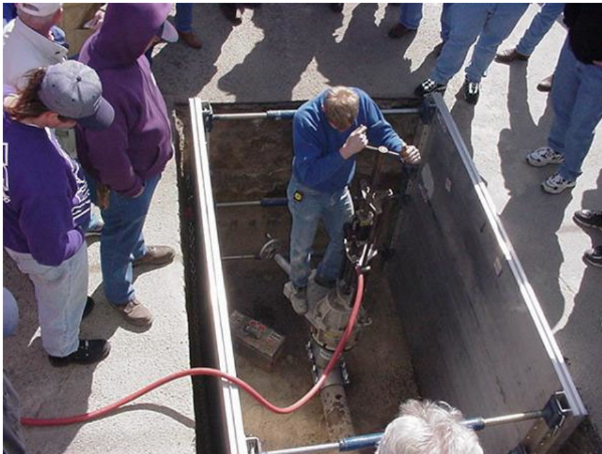
Hydro-Stop valve insertion machine
