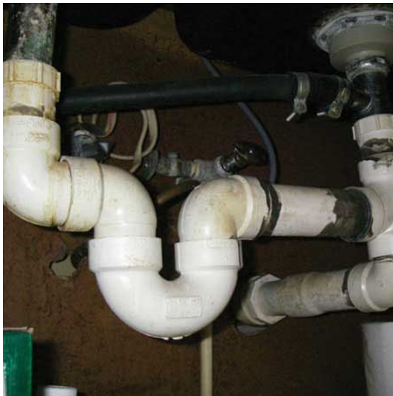
Top photograph, never install electricity near a water outlet. Bottom, there's room here...let's put the u-trap here. NOT!
