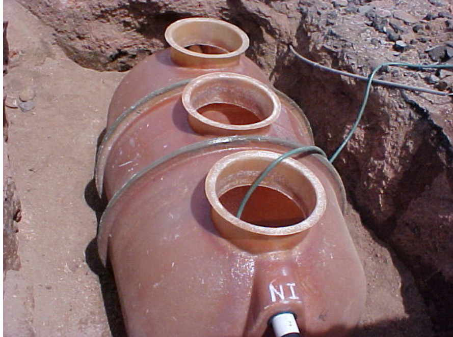
Three Compartment Grease Interceptor
