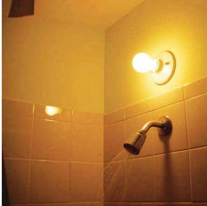
Top photograph, never install electricity near a water outlet. Bottom, there's room here...let's put the u-trap here. NOT!
