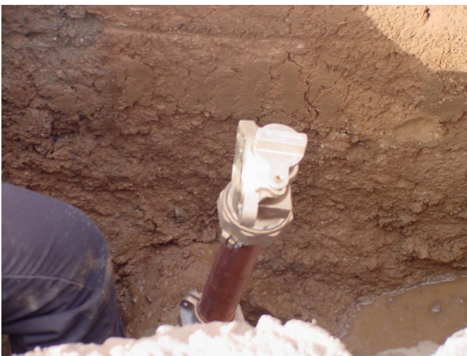
Installation of a new customer water service line.
