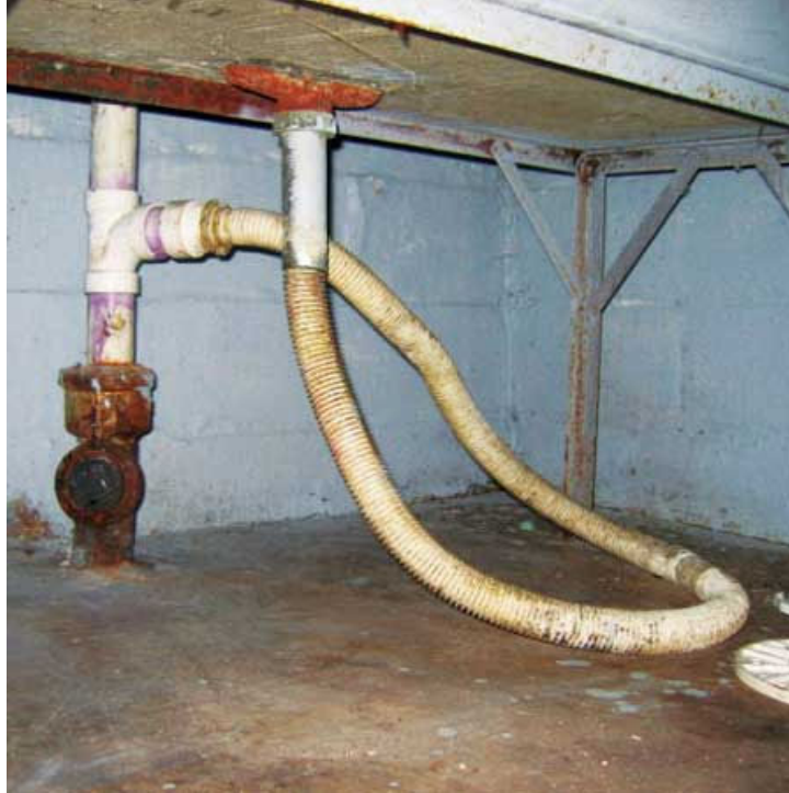
Top photograph, no trap needed when you have a long flex hose. Bottom, this is a new side trapper. NOT!
