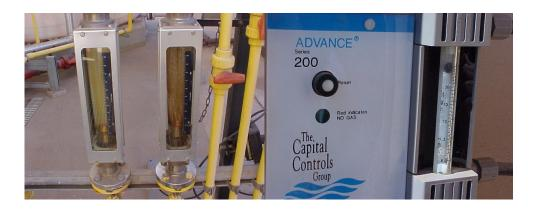
Chlorine measurement devices or Rotameters.
