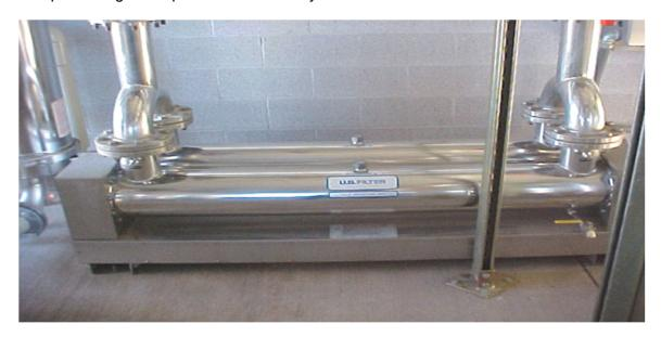
The lamp itself does not come into direct contact with the water, The lamp is placed inside a quartz tube, and the water is in contact with the outside of the quartz tube. Quartz is used in this case since practically none of the UV rays are absorbed by the quartz, allowing all of the rays to reach the water.
