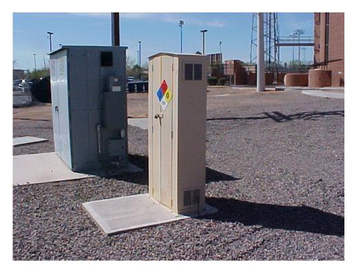
Small chlorine storage shed in the foreground; notice the vents at the bottom and top. The bottom vent will allow the gas to ventilate because  $\text{Cl}_2$  gas is heavier than air.
