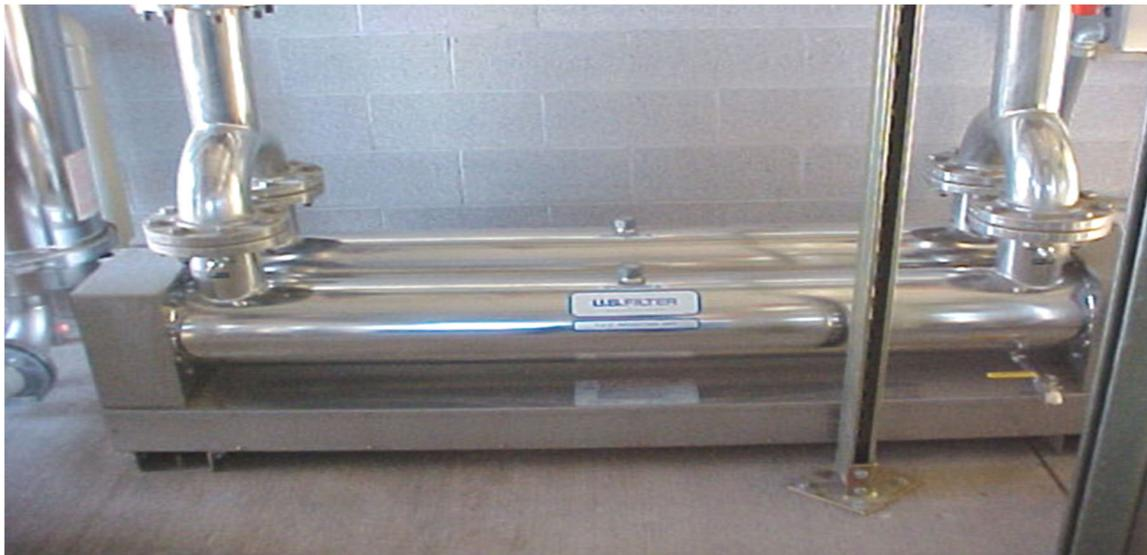
The lamp itself does not come into direct contact with the water, The lamp is placed inside a quartz tube, and the water is in contact with the outside of the quartz tube. Quartz is used in this case since practically none of the UV rays are absorbed by the quartz, allowing all of the rays to reach the water.
