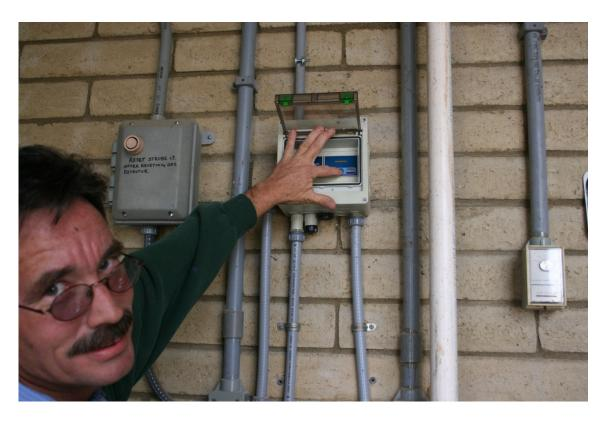
Top photograph, adjusting the Chlorine leak alarm sensor. Bottom photograph, Chlorine container weight scales.
