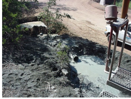
Constructed Mud Pits
