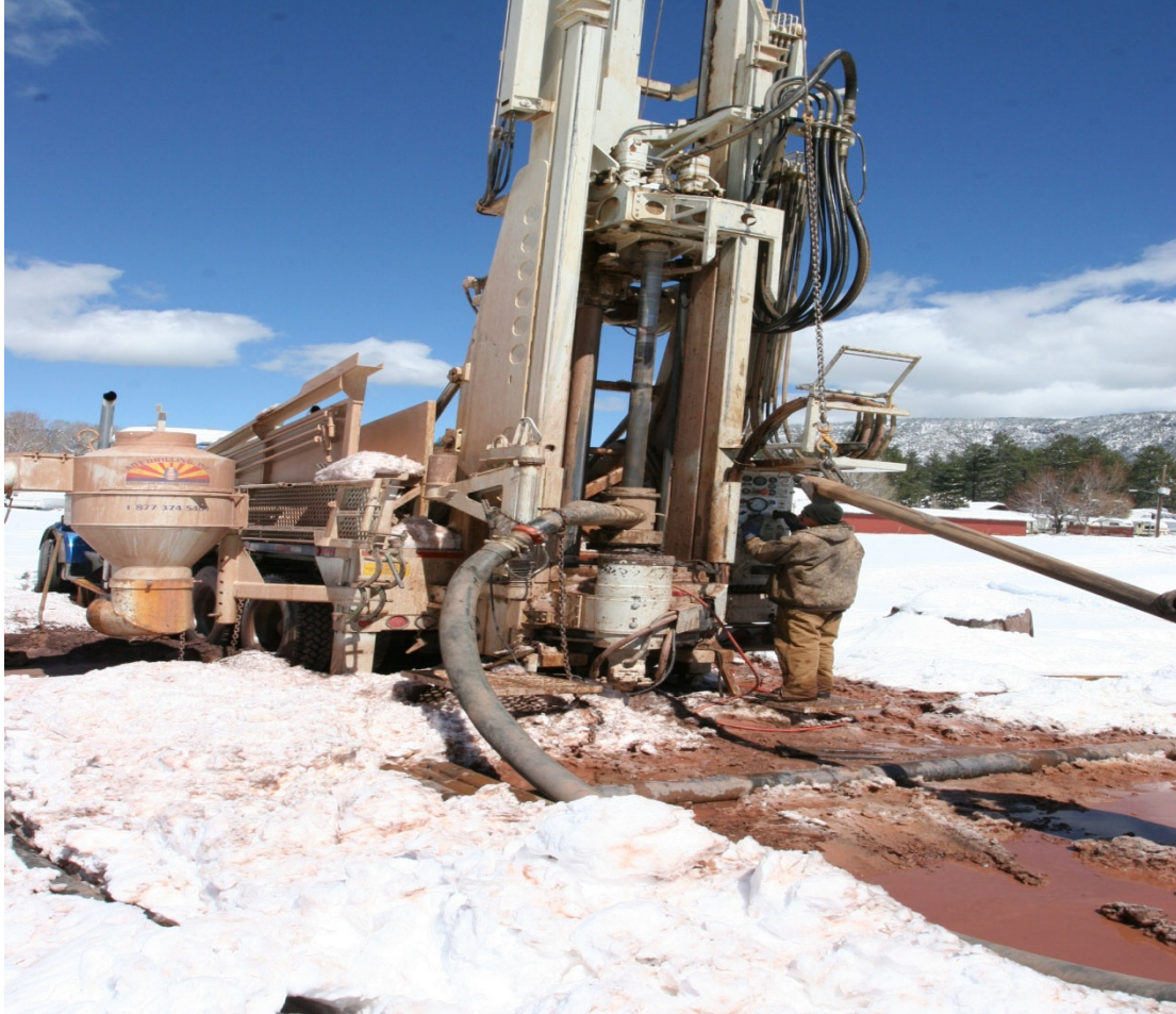
A drill rig in the snow.
