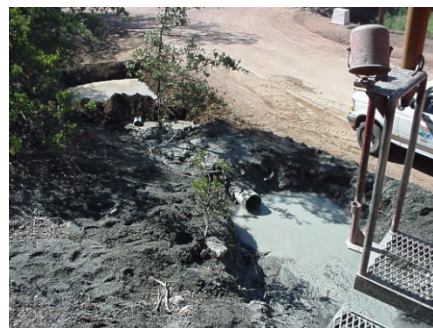
Constructed Mud Pits
