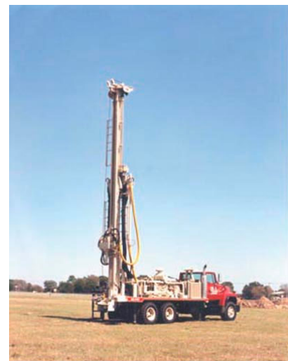
Typical Rotary Rig
