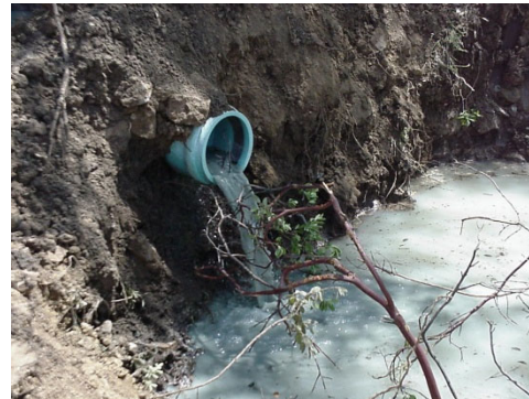
Last Pit (small amount of fines)
