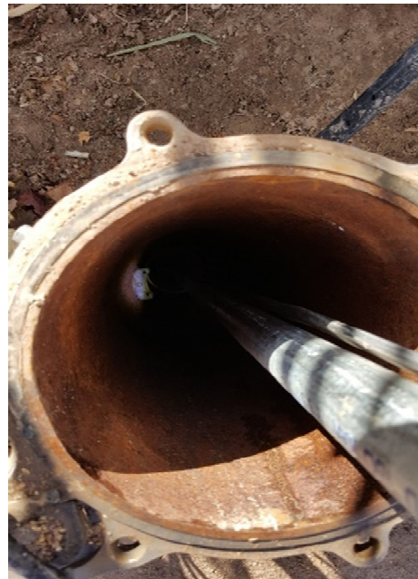
Well cap removed, looking at pvc pipe and electrical wire
