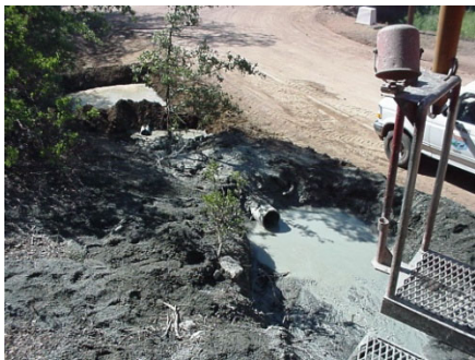
Constructed Mud Pits
