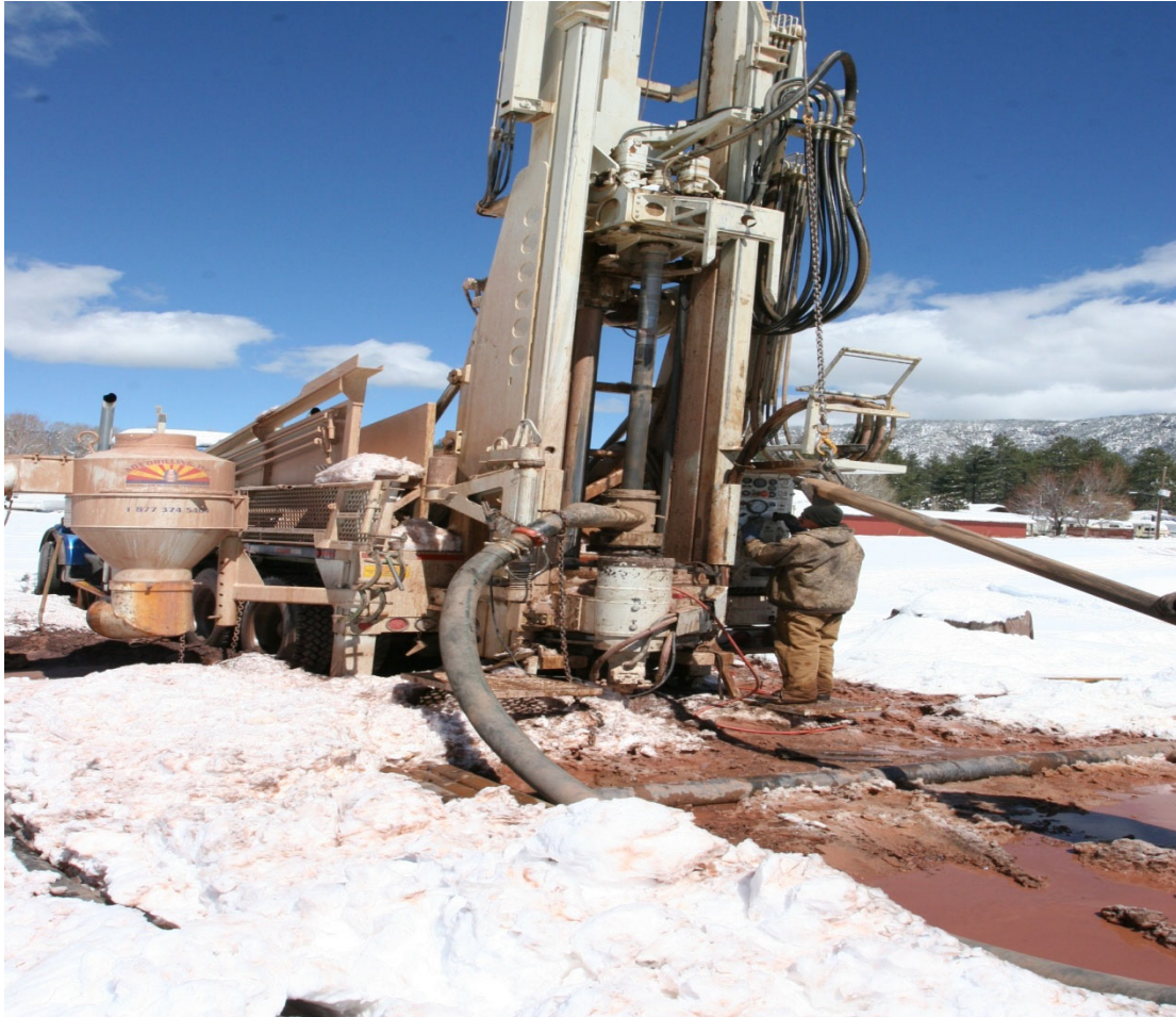
A drill rig in the snow.
