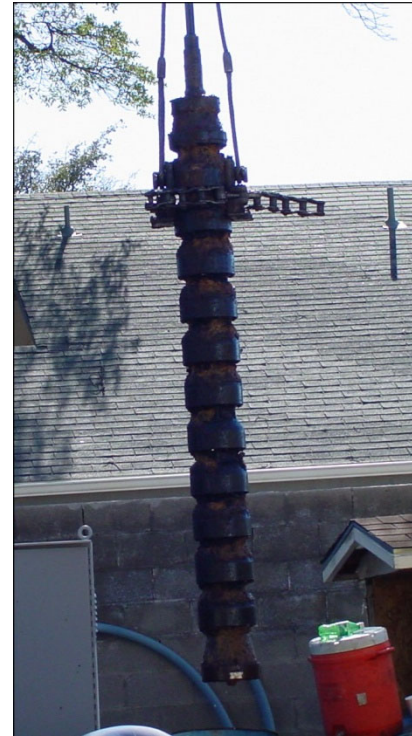
Above, Vertical Turbine Pump Being Removed (notice line shaft)
