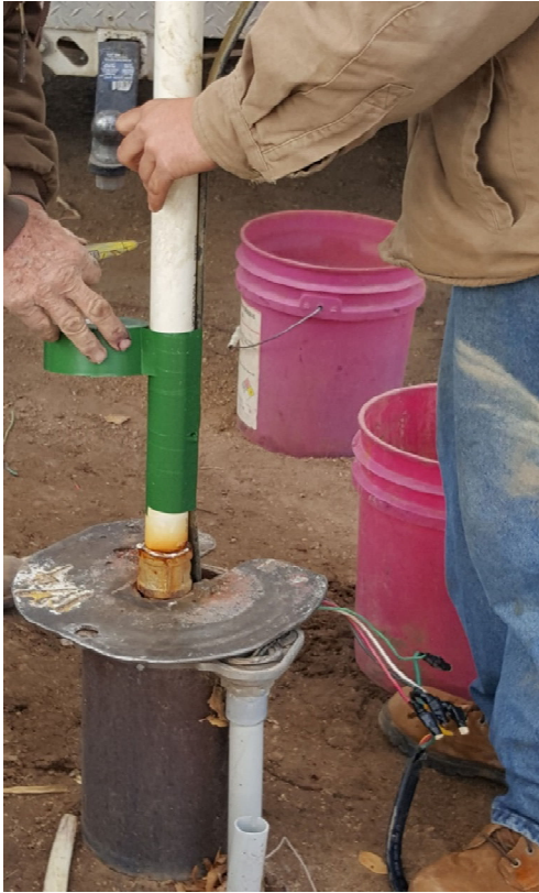
Installing new submersible pump, securing wire and connecting pump wiring.
