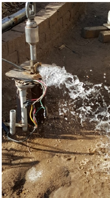
Installing new submersible pump, securing wire and connecting pump wiring.
