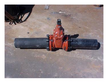
Here a Gate Valve is prepared for a valve replacement.
