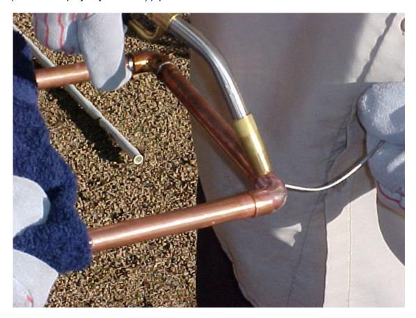
Soldering pipe, there are several types of copper pipe. Soft and rigid, K-Green, L-Blue, M-Red, and DWV-yellow. You can no longer use lead solder for potable water. Copper lines fit together with lead-free, solid-core solder. The soldering process involves heating the pipe and is commonly called "sweating."
