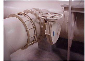
The valve should be installed in the closed position to ensure that the laminated seal in the disc is not damaged during installation.
