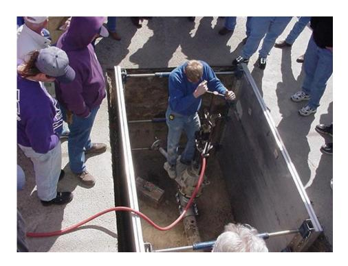
Hydro-stop valve insertion machine
