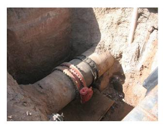
54 inch Butterfly valve on a huge transmission line. Nice job but no shoring, no ladder or valve blocking.
