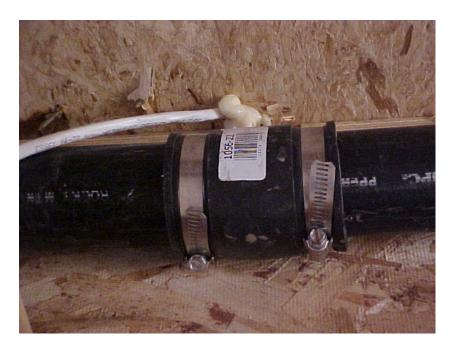
No Hub compression type fitting used on drain, waste and vent lines.
