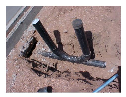
2-Way Cleanout DWV Soil Pipe, needs to be within 2 feet of the house, perpendicular (not parallel) to the footing and the end or grade level needs to be painted to protect from sunlight.
