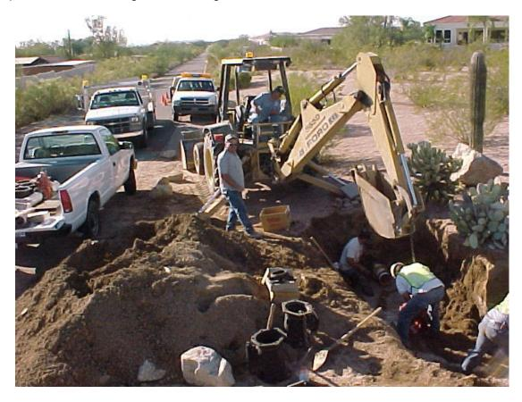
Repair crew replacing three tapping valves that blew out during a leak.
