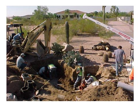
Top photograph, two gate valves blew out, you can see the kickers or thrust blocks in the back ground. Bottom photograph, a tapping machine and a new gate valve. These tapping machines are very expensive.
