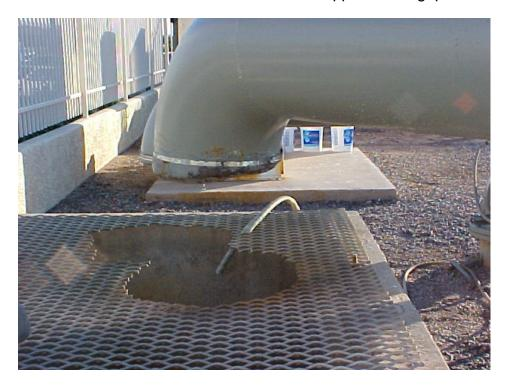
Notice the larger pipe is an approved air gap, but what about the smaller drain in the rear?
