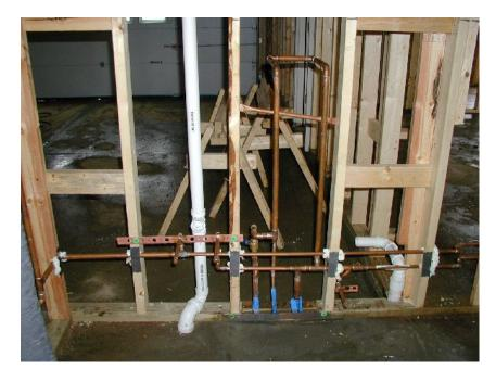
Lavatory or bathroom set-up with a Dirty Arm and possible water softener loop.
