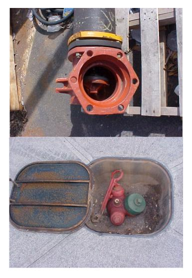
Bottom of a dry barrel fire hydrant--there is a drainage hole on the back of this hydrant, sometimes referred to as a "weep hole". Below is an "Airport Runway" type of hydrant.
