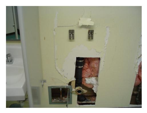
Prepare for extensive wall damage when retrofitting to a waterless urinal. You may need to replace tiles and drywall. Notice the square box on the right hand side, this is a trap primer for the floor drain. The trap primer keep a small amount of water to keep the drain's trap wet to prevent sewer odors from coming up.
