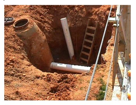
Sewer lateral going into a manhole.
