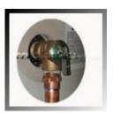
All domestic water heaters are required to be equipped with a relief valve as a safety
