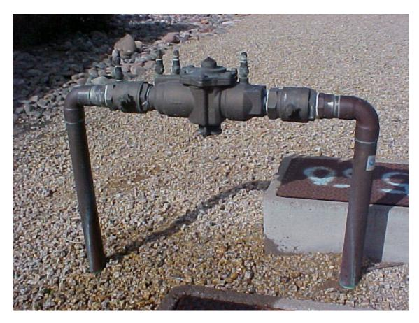
Leaky RP probably has some debris in the pressure differential area or in the hydraulic relief valve area.
