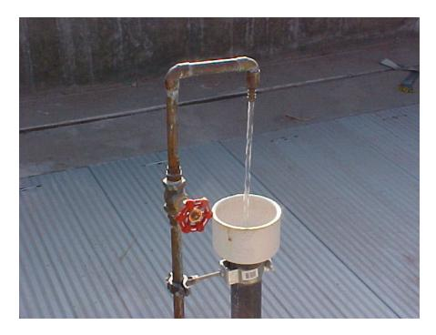
**Sample Station commonly found at most water or wastewater treatment plants.** This tap will allow the operator to obtain Grab Samples for pH, Temperature, COD, Bacterial, ORP, OUP, Organics and Inorganic field parameters.
