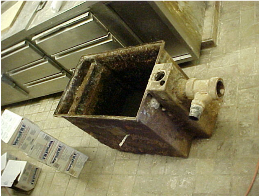
In-floor Grease trap being removed and replaced with a grease interceptor. Unfortunately, most grease traps are not properly maintained.
