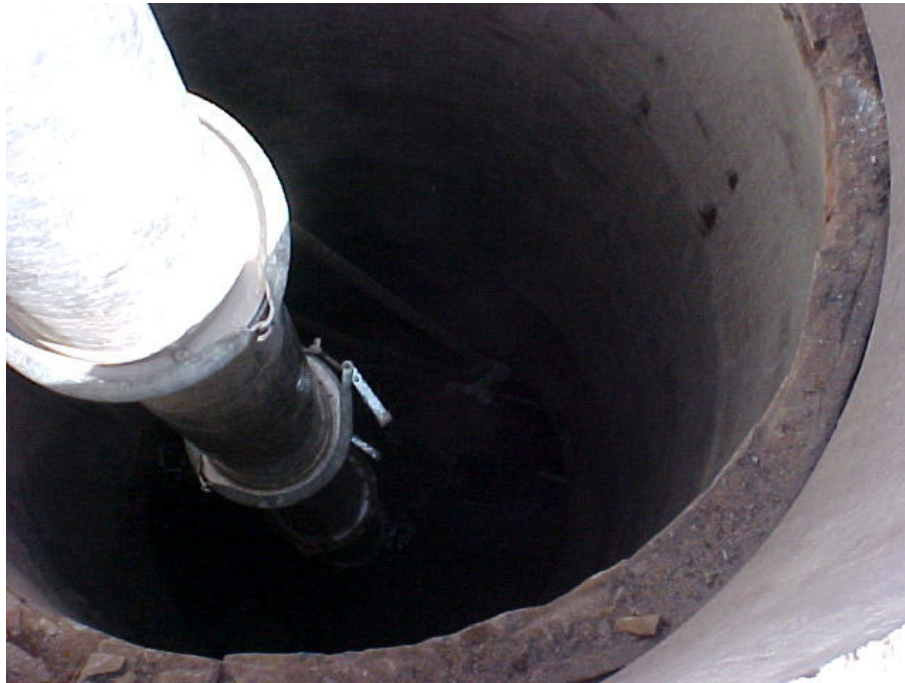
A Vactor clearing a Manhole.
