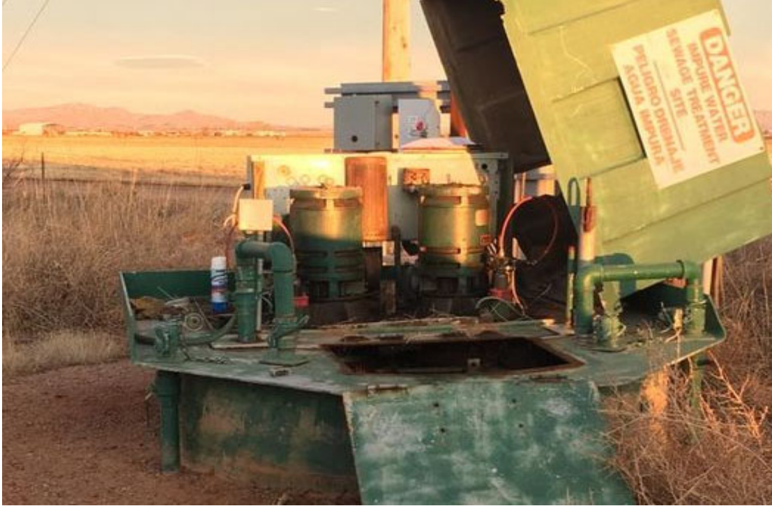
Top photo, Centrifugal pump is the most common wastewater lift station pump. Bottom photo, A trapped air column, or bubbler system, that senses pressure and level is commonly used for pump station control.
