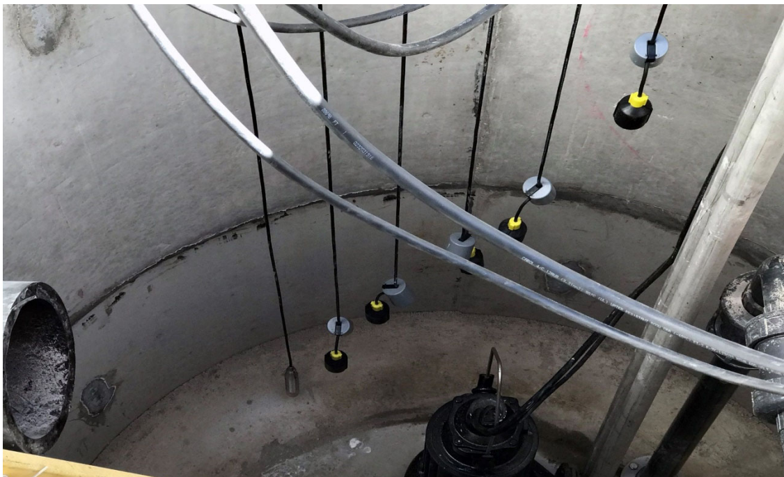
Top photo, Centrifugal pump is the most common wastewater lift station pump. Bottom photo, A trapped air column, or bubbler system, that senses pressure and level is commonly used for pump station control.
