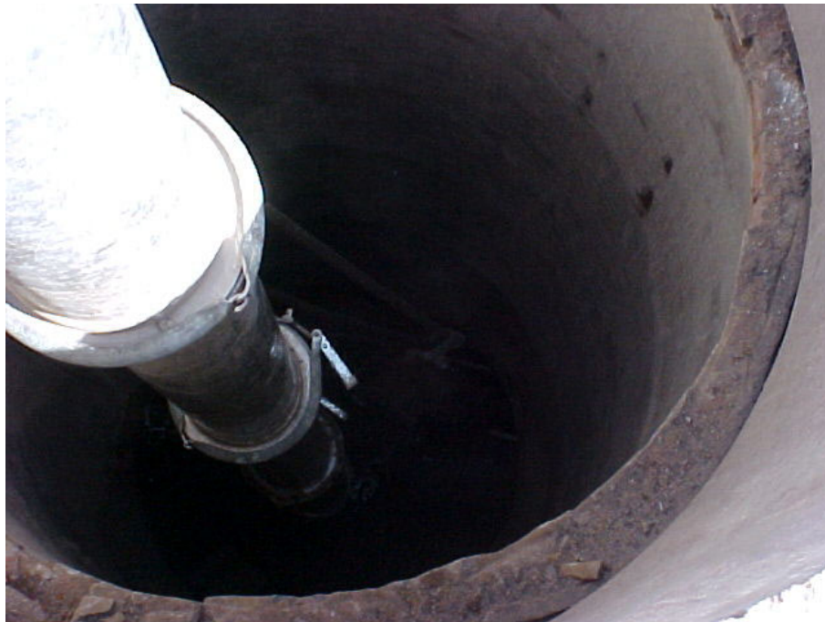
A Vactor clearing a Manhole.
