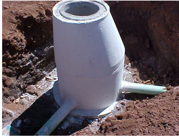
Newly finished Manhole and Laterals
