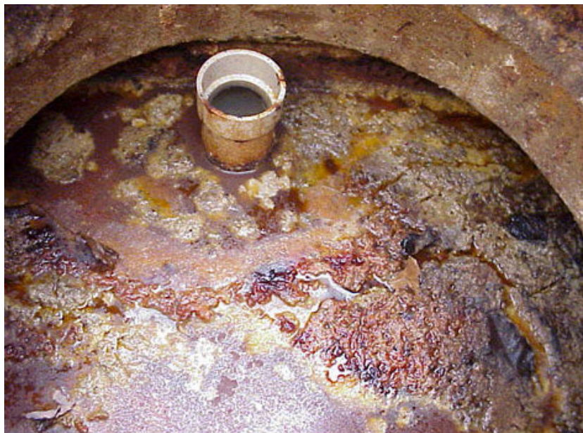
Looking down into a grease interceptor commonly used in a commercial food service operations.
