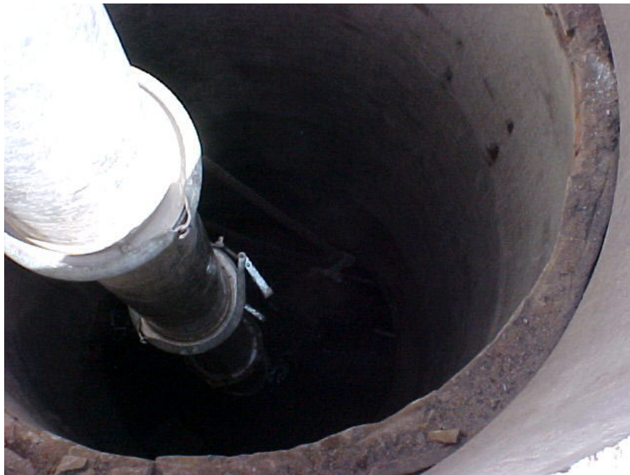
A Vactor clearing a Manhole.
