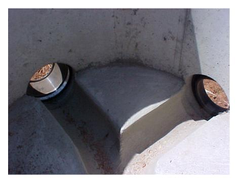
Inside a new manhole, the Invert is the inside bottom of the pipe. The Invert is used to determine the depth which is used to determine the Rise or Slope of the pipe.
