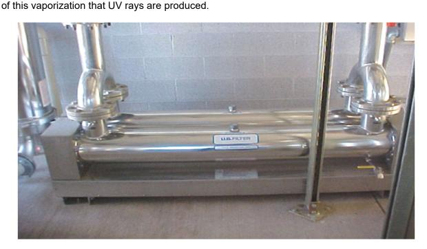
Enclosed UV lamp assembly. Assemblies will often need frequent cleaning and bulb replacements, there are facilities with 1,000's of bulbs.
