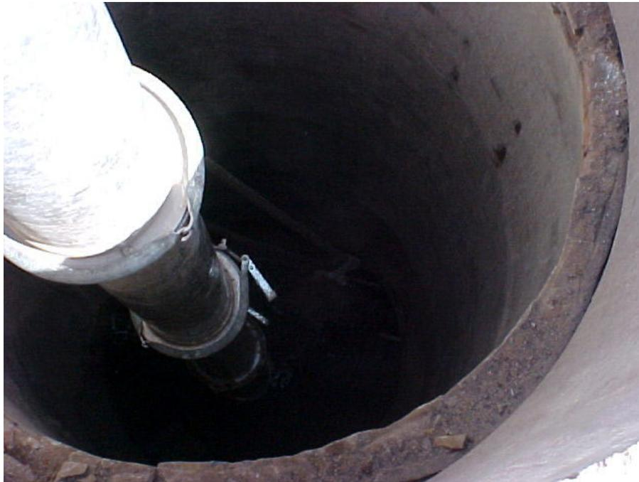
A Vactor clearing a Manhole.
