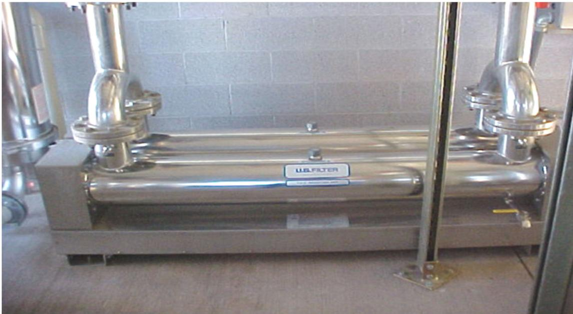
Enclosed UV lamp assembly. Assemblies will often need frequent cleaning and bulb replacements, there are facilities with 1,000's of bulbs.
