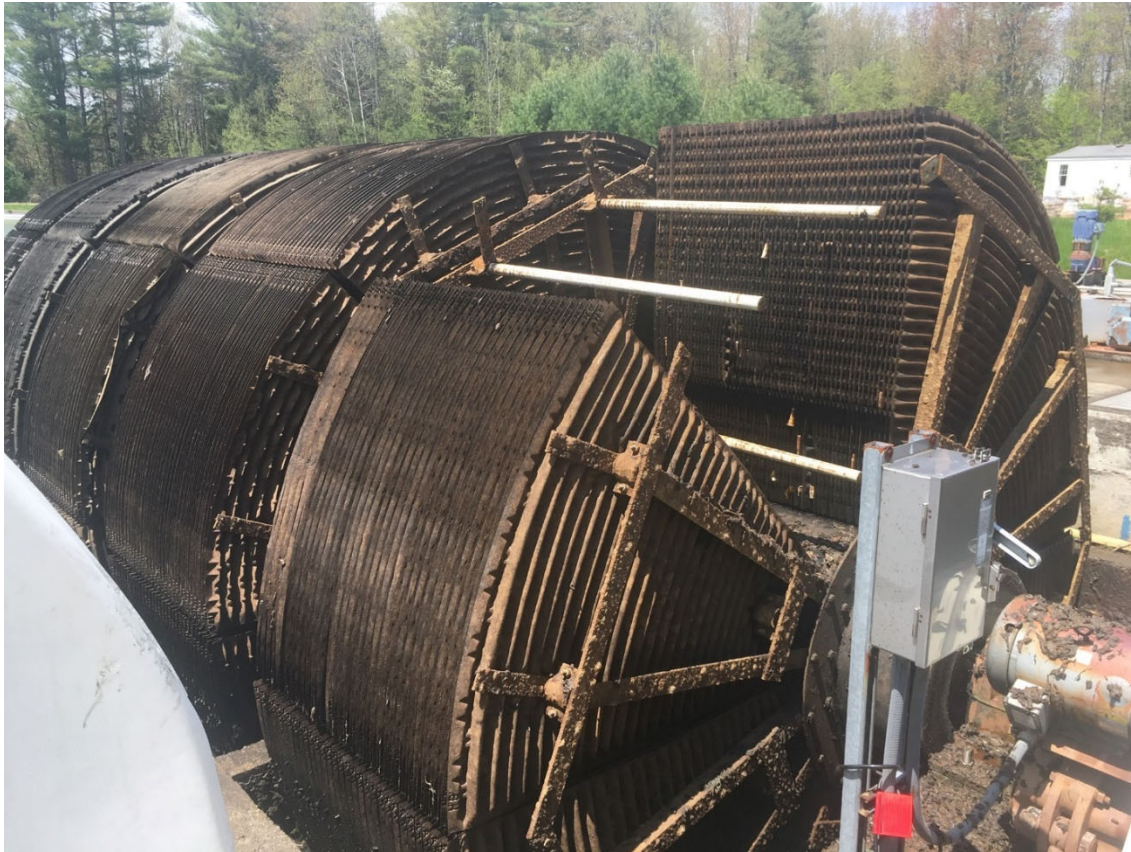
An RBC with one section removed.
