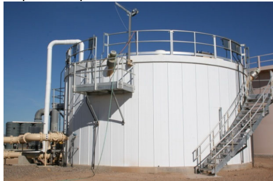
Anaerobic Digester
