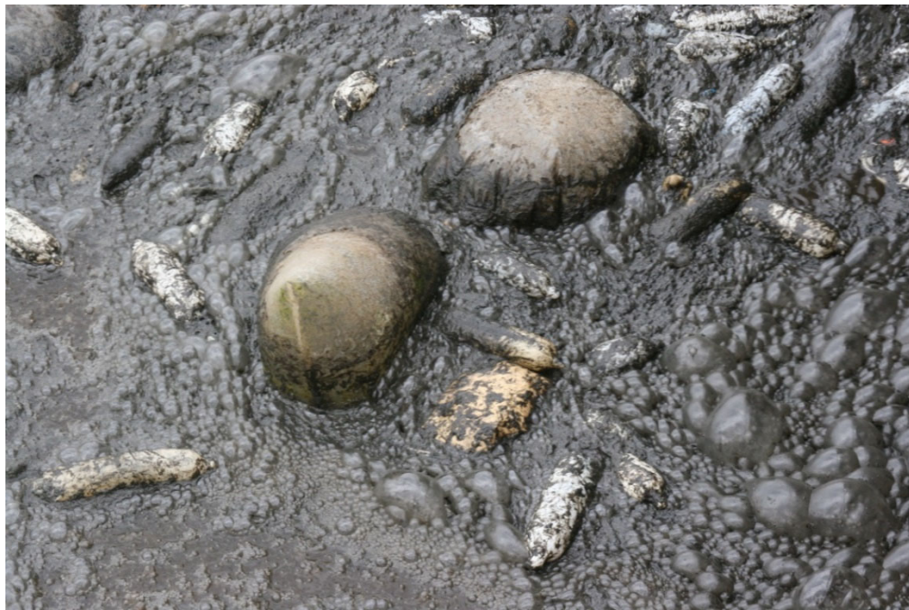
Floating scum in an influent chamber. This debris should be removed and sent to a landfill.
