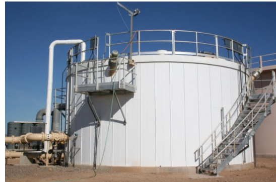
Anaerobic Digester
