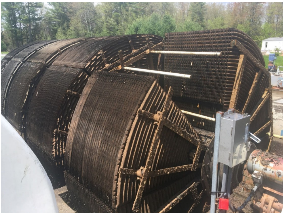
An RBC with one section removed.
