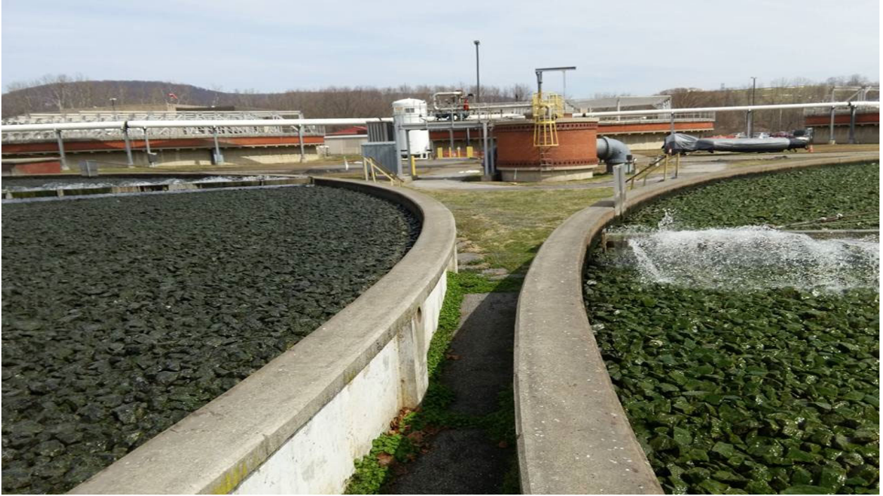
Fixed-film trickling filters. The left filter discoloration is due to sloughing. The photo below is the actual material off that filter.
