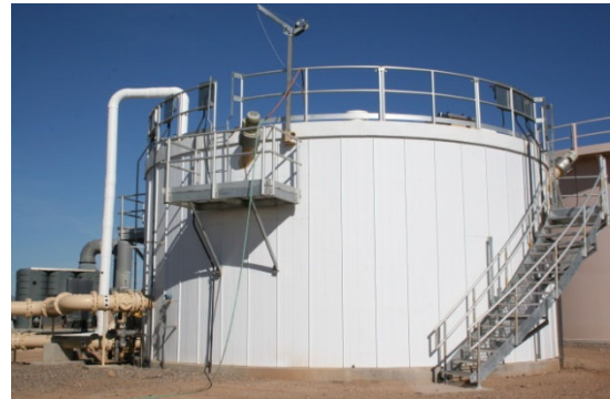
Anaerobic Digester
